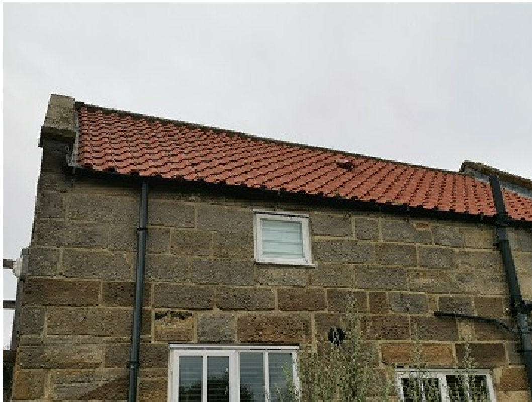
Plate 8. Shows east elevation of Building 3
