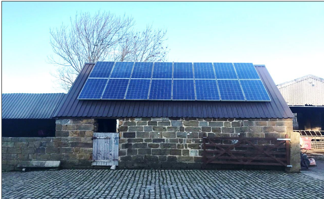
Photo 1. The surveyed building.
