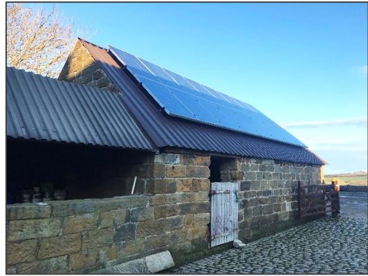
Photo 3. West and south aspects.
