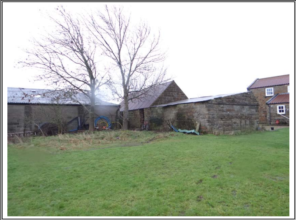
Photo 1 General view of the barn from the farm house garden to the north west.
