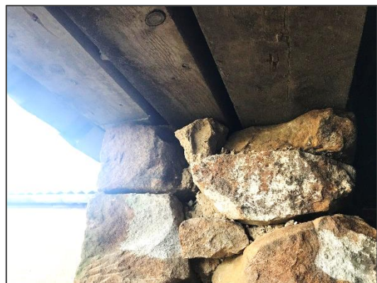
Photo 9. Masonry/lintel crevices.
