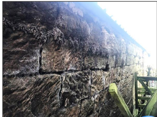
Photo 7. Masonry crevices.
