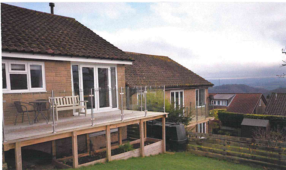
Further photograph of the rear which shows the dormer to no 16 which has a similar section to that proposed.
