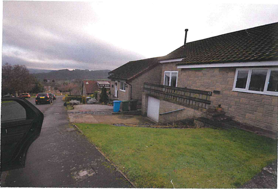
Photograph of the front of the property again showing the fairly recent dormer to no 16.
