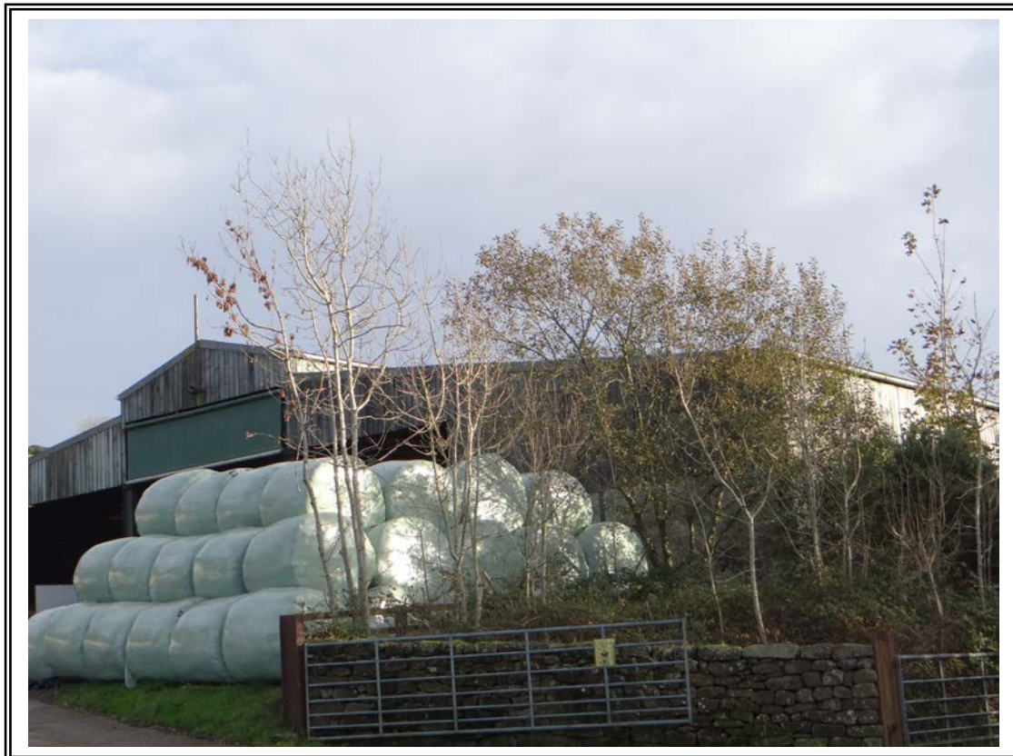
Photo 2 North west corner of the existing shed. Note the silage bales are where the extension is proposed. Trees will be retained for screening.
