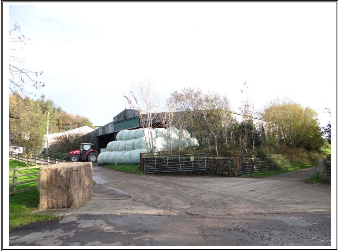
Photo 4 View of the shed from the road. Note trees to be retained.
