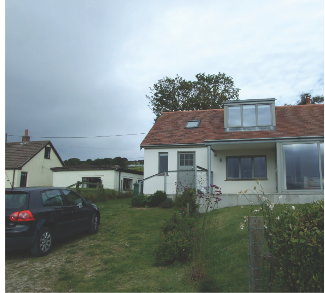
Crestbank - Existing render to front elevation photograph
