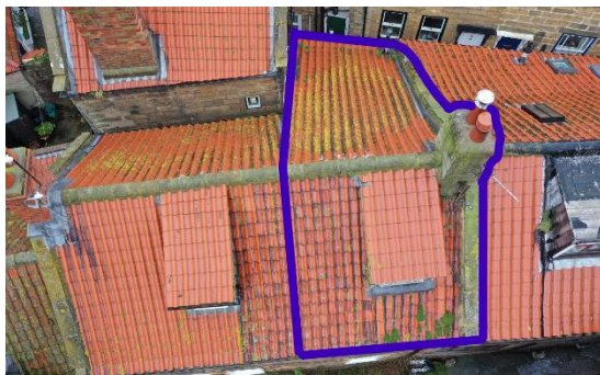
Image of existing roof
