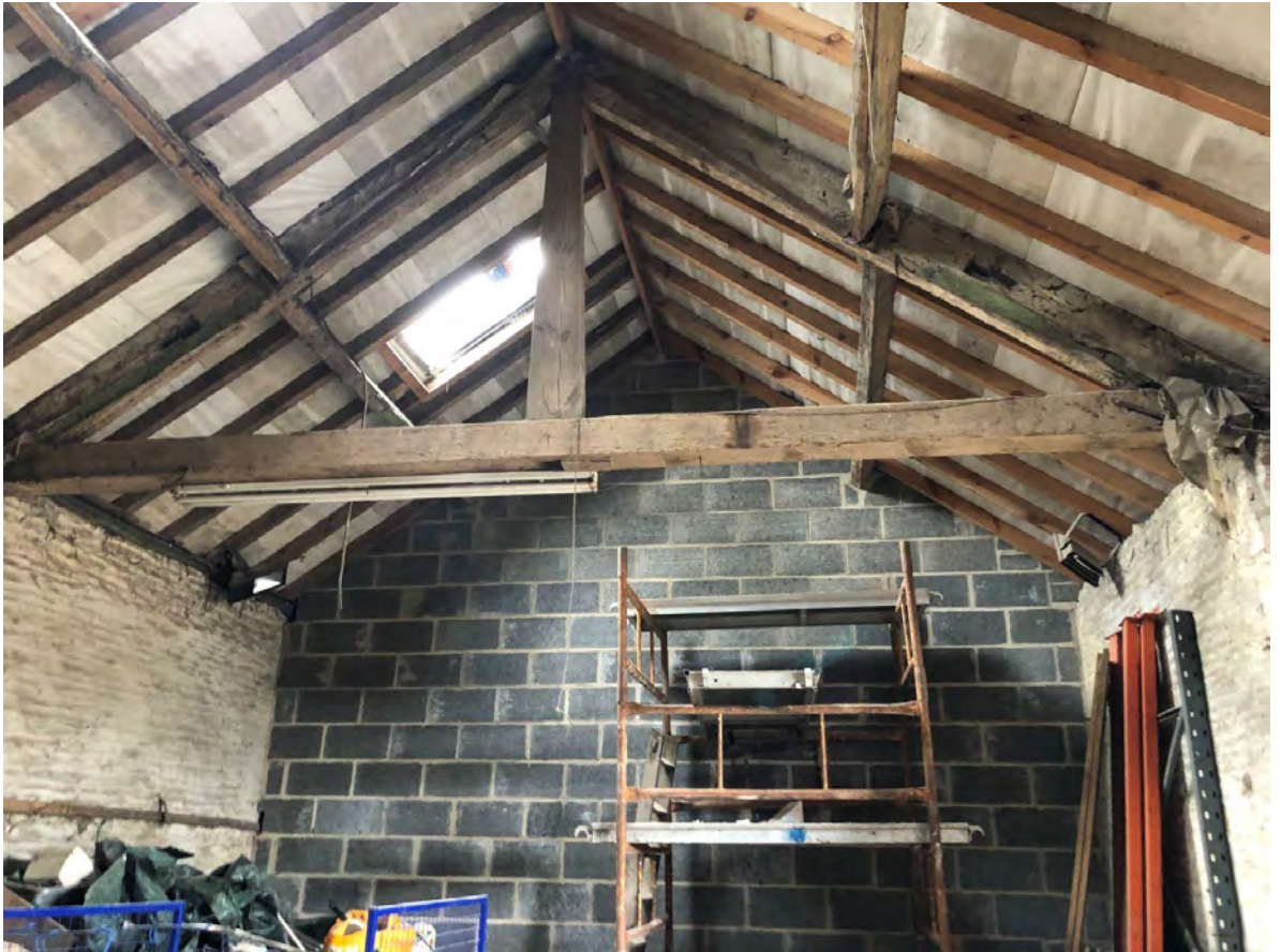
Photograph 2 Existing Roof Truss
