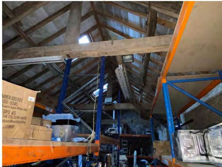
Plate 4 – barn, internal roof void.
