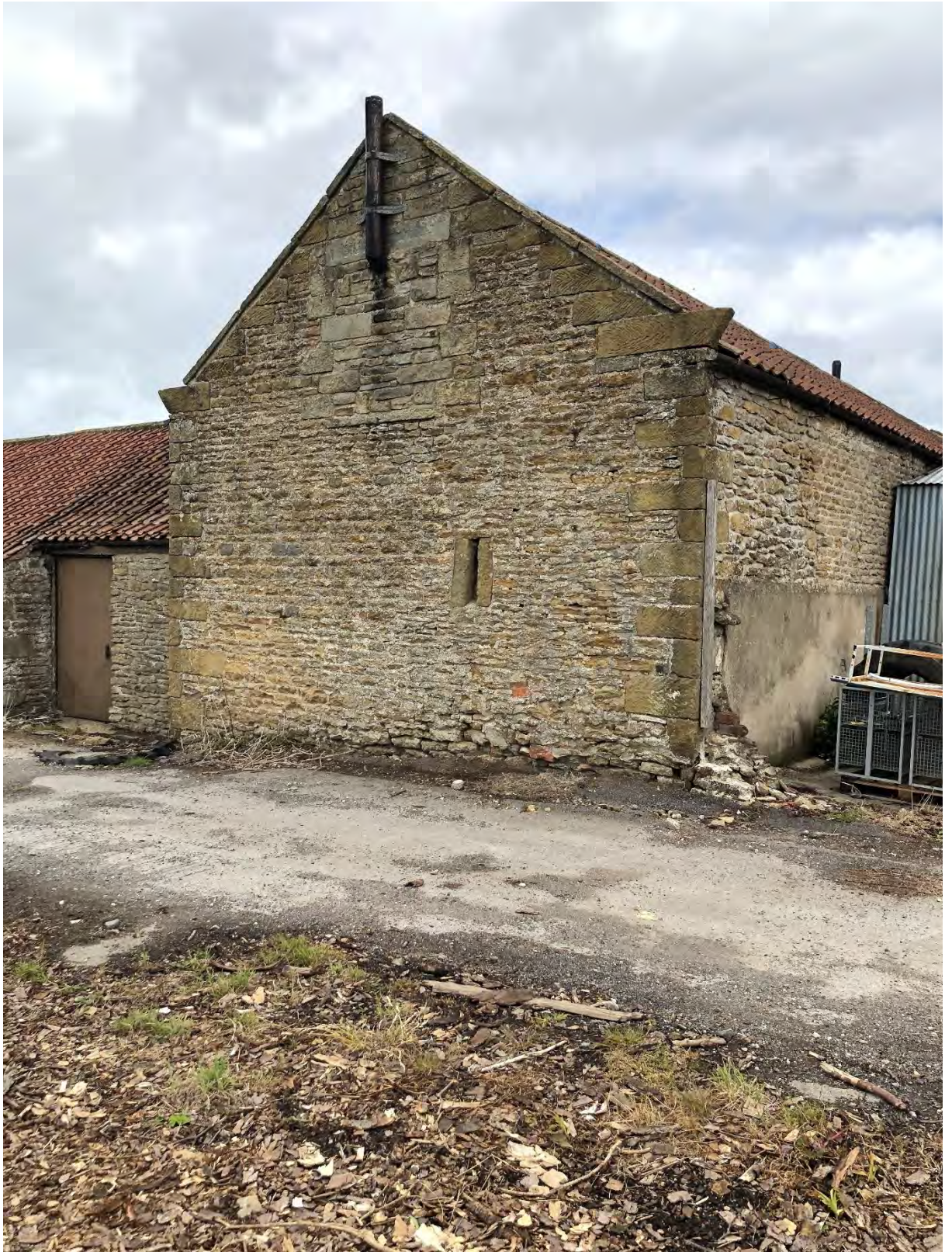
Photograph 3 South gable with outline of previous opening visible
