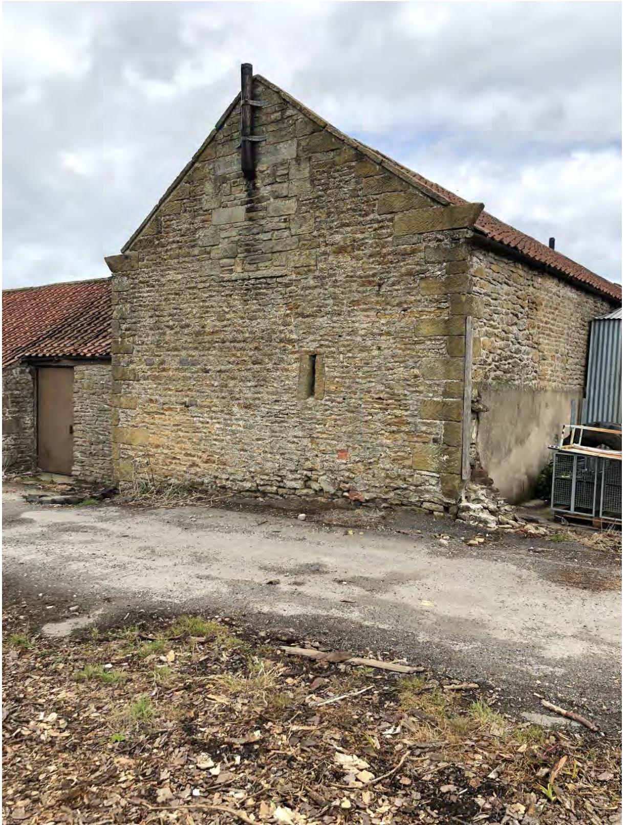
Photograph 2 South gable elevation
