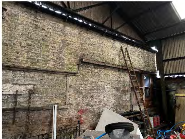
Plate 3 – barn, west elevation.
