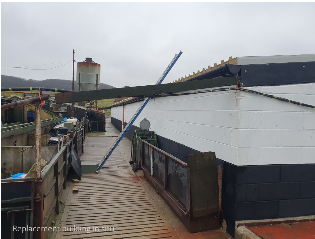
Replacement building in situ
