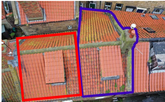
Image of existing roof
