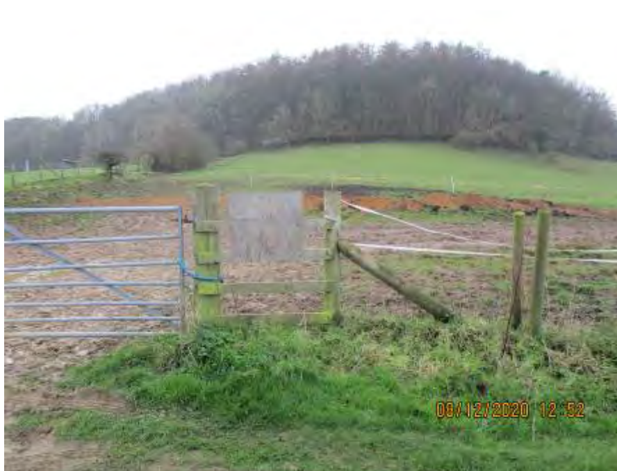
Image showing the earth works that have been undertaken in connection with the drainage works
