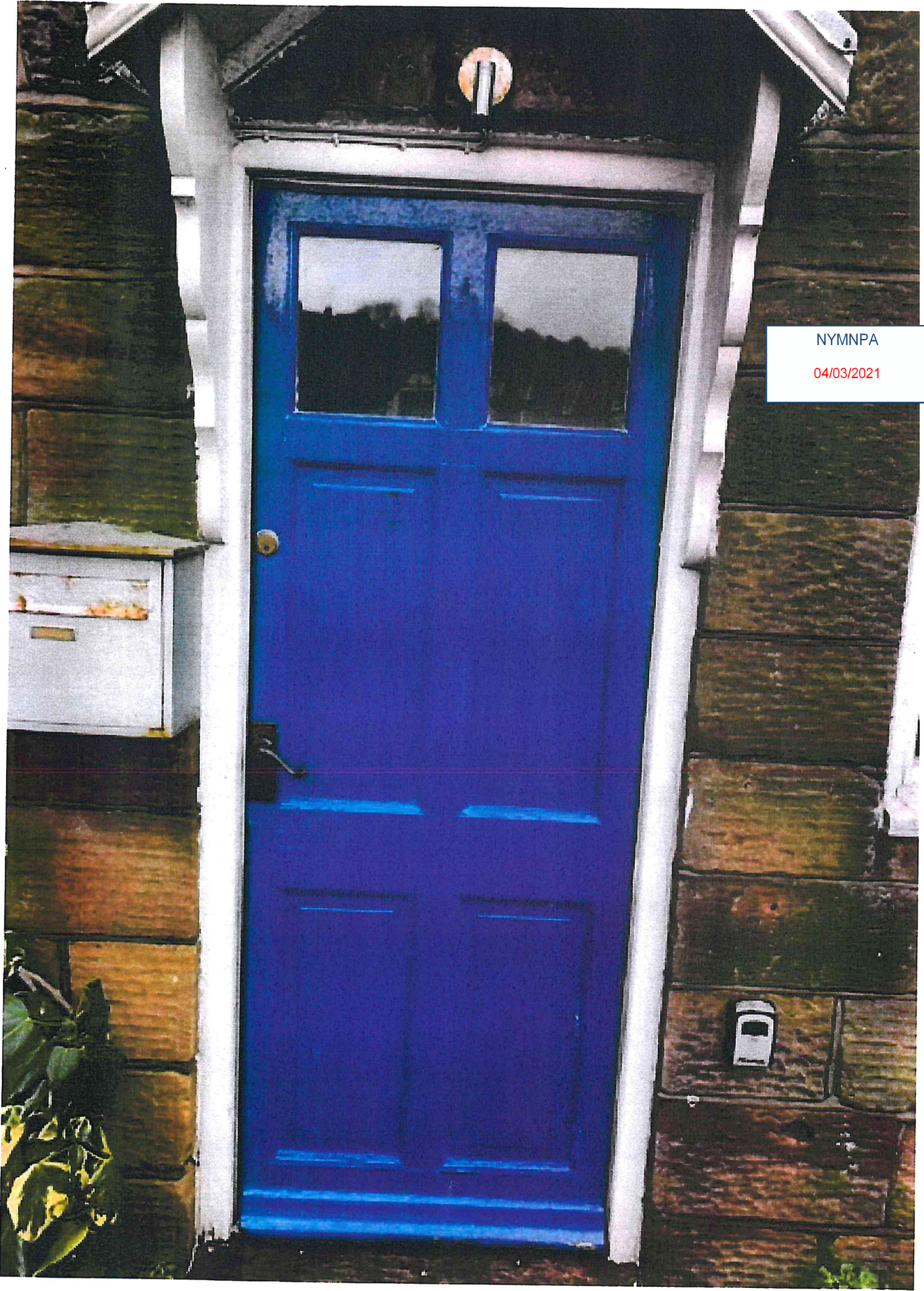
EXISTING FRONT DOOR
