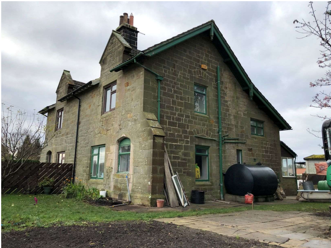
Side (east) Single storey rear extension to 2 Railway Cottage, Goathland, YO22 5LY
