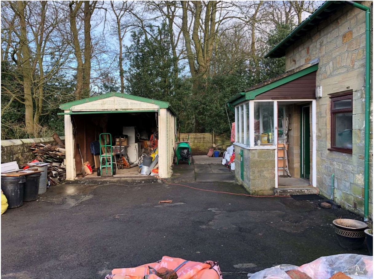
Photograph 3 View from the south elevation
