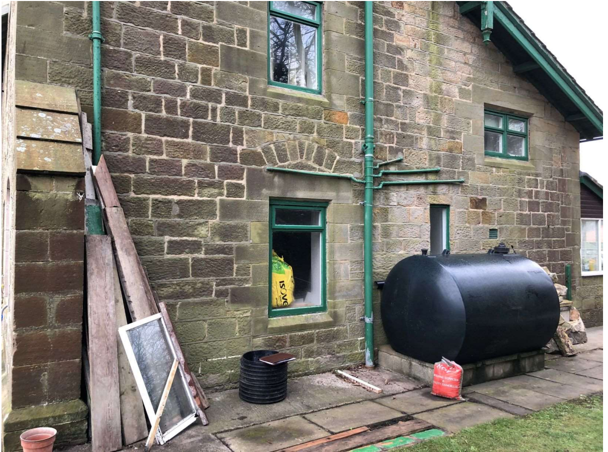
Photograph 1 Existing side elevation
