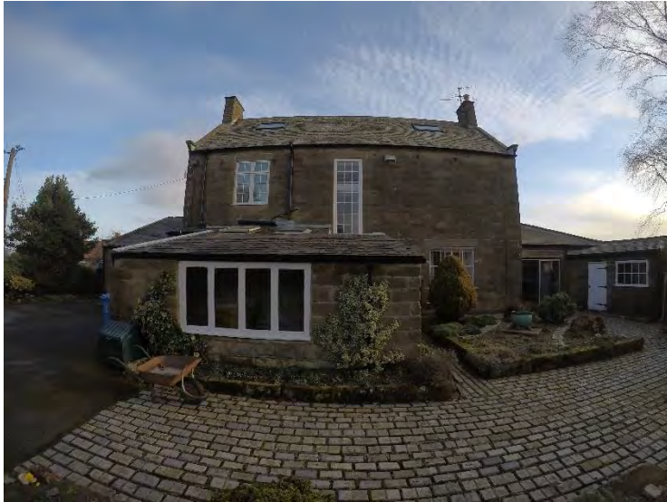
Photo 8: Rear of house, showing existing paved setts
