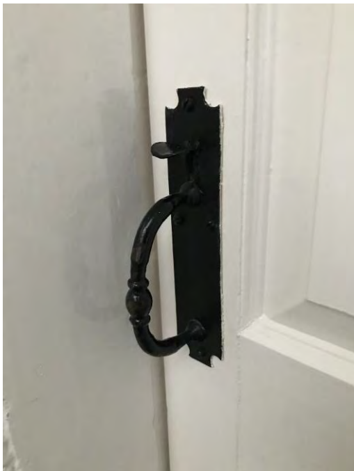
Photo 58: Rear Corridor door latch
