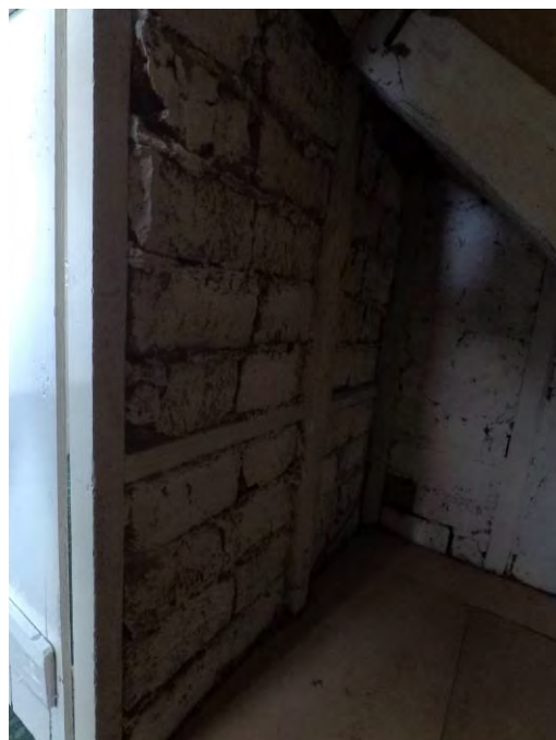
Photo 48: Cupboard interior with brick panels
