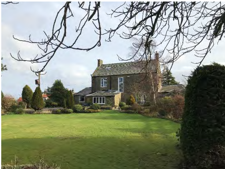
Photo 12: Rear of house viewed across garden from shed
