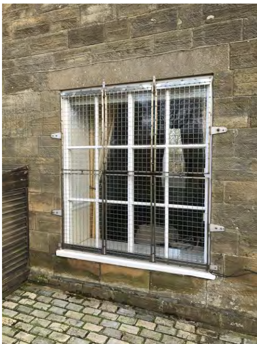
Photo 65: Rear window to Living Room
