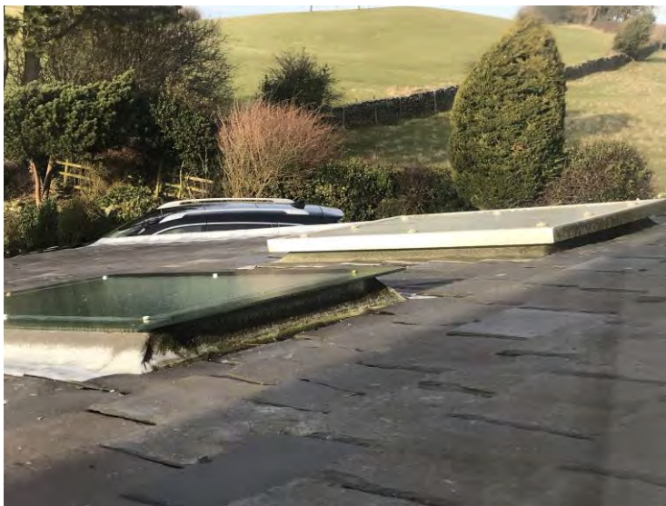
Photo 62: Rooflights over Rear Hall and Utility Room
