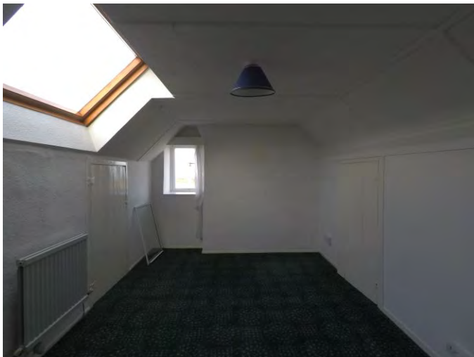
Photo 46: Bedroom 5 looking east
