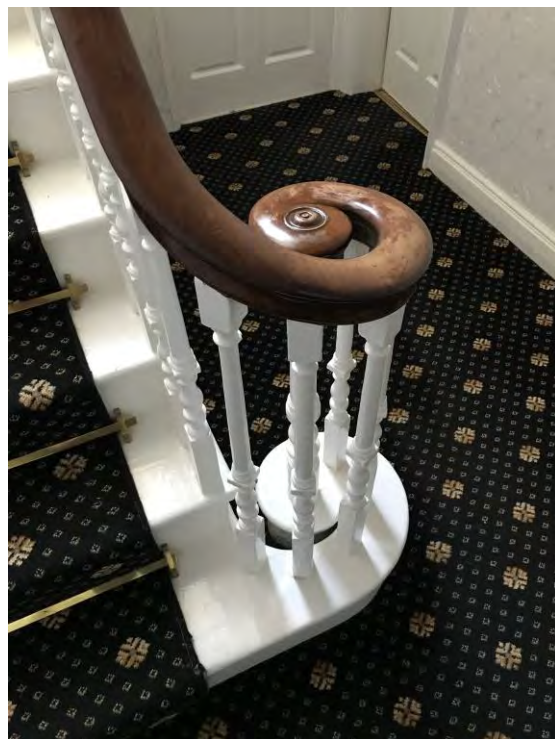
Photo 30: Stair handrail detail
