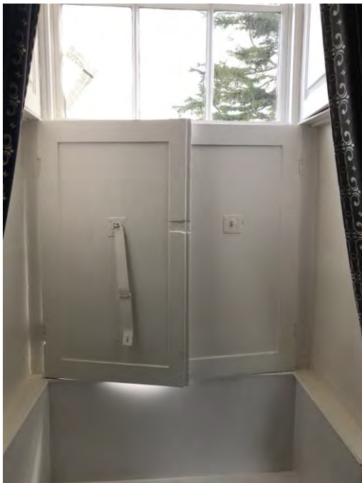
Photo 54: Closed shutter panels (where window set in deep reveal)
