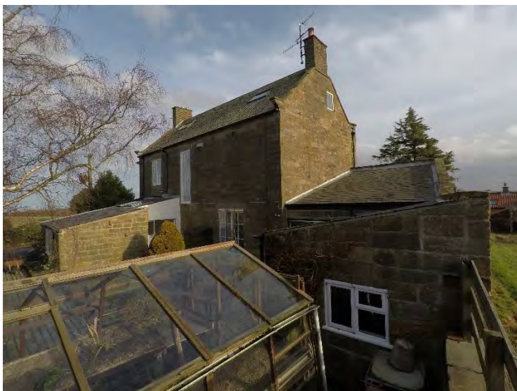
Photo 10: Rear of house, showing existing greenhouse
