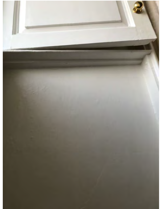
Photo 53: Window shutter box
