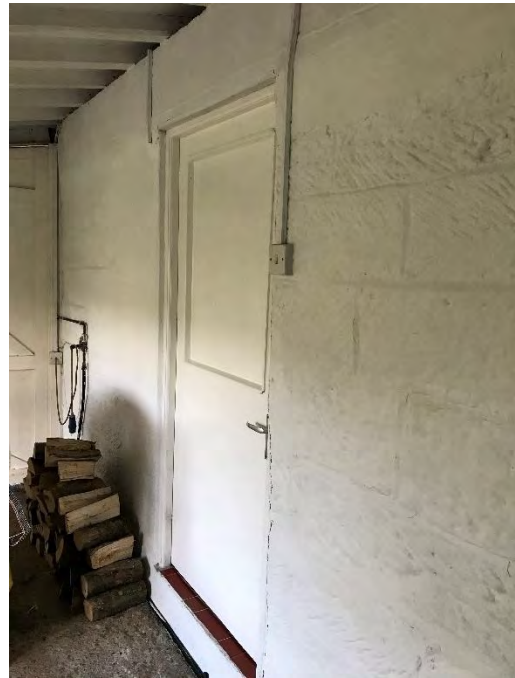
Photo 19: Rear wall of Utility in Garage
