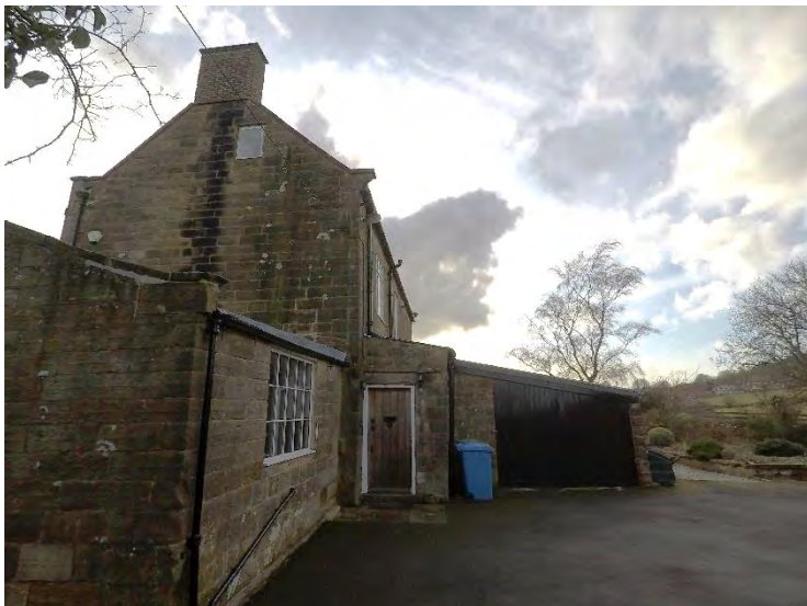
Photo 6: Rear Entrance Door viewed from east
