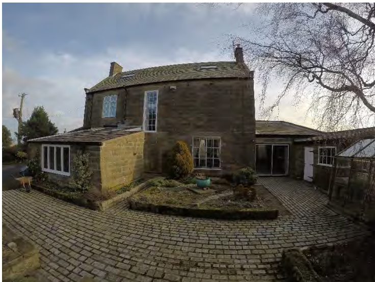
Photo 9: Rear of house, showing existing paved setts
