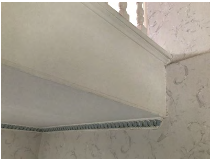
Photo 51: 1 st Floor Landing Cornice
