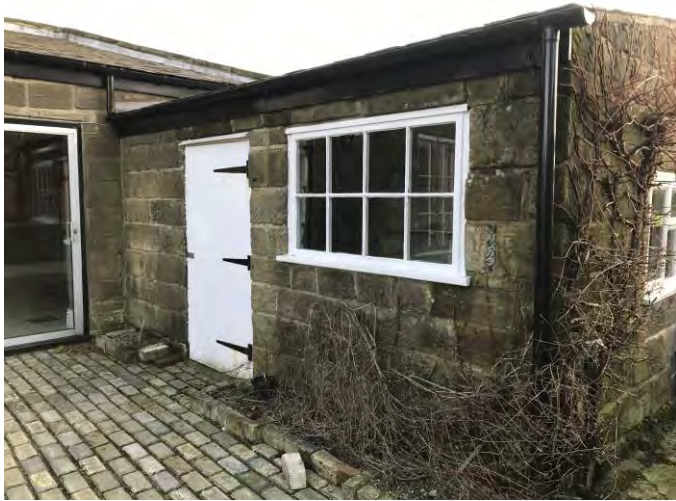
Photo 63: Outbuilding abutting rear of building on western boundary
