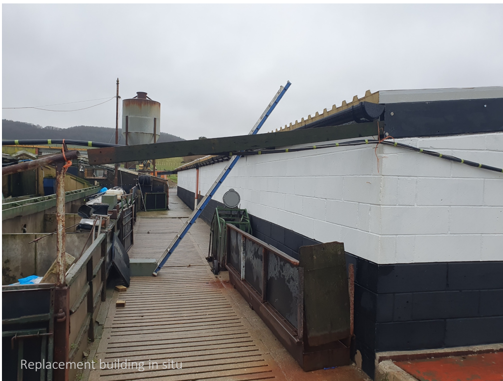
Replacement building in situ
