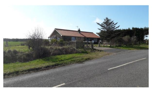
Photograph of Fir Tree Lodge taken from the road. The property is a linear bungalow, orientated parallel with the road of random stone construction under a red pantile roof with central chimney stack and small lean-to porch on side (gable elevation). It is set back in the plot with timber post and rail fence boundary with fir trees to the north (right) boundary and an open pasture field to the south (left).
