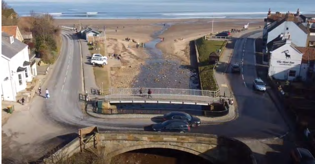
Figure 1 – Example of two-way flow over East Row Bridge
