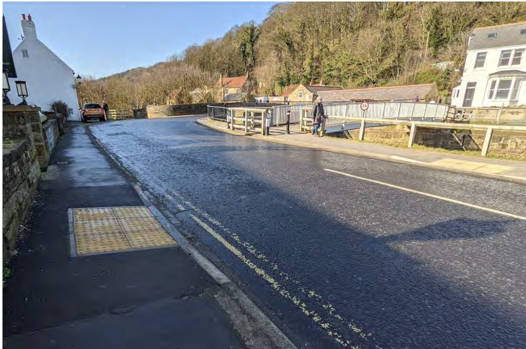
Figure 2 – Photo of existing infrastructure in proximity to East Row Bridge
