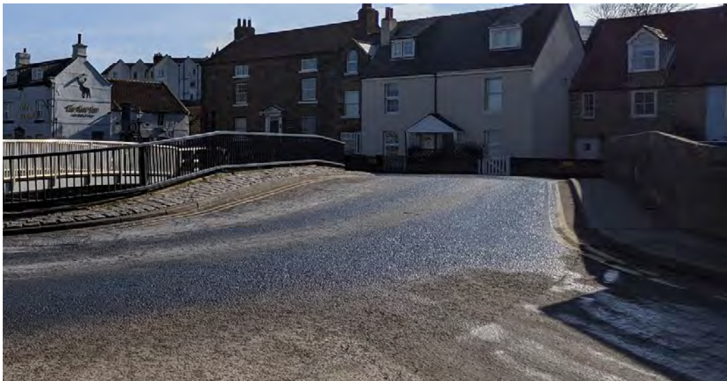
Figure 3 – Photo of existing pedestrian deterrent paving
