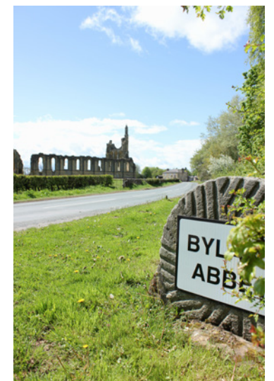
The abbey church north elevation from the Wass to Coxwold road.
