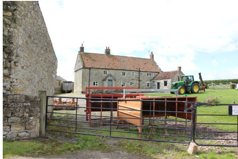
College Farmhouse, Grade II listed as seen from the Byland Abbey to Olstead road
