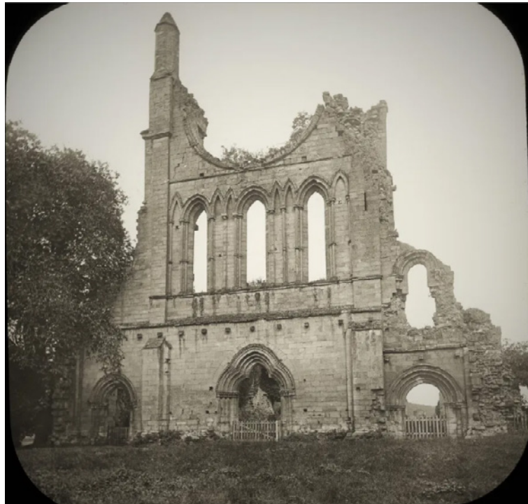
An early photograph of the west front before the site was taken into state care
