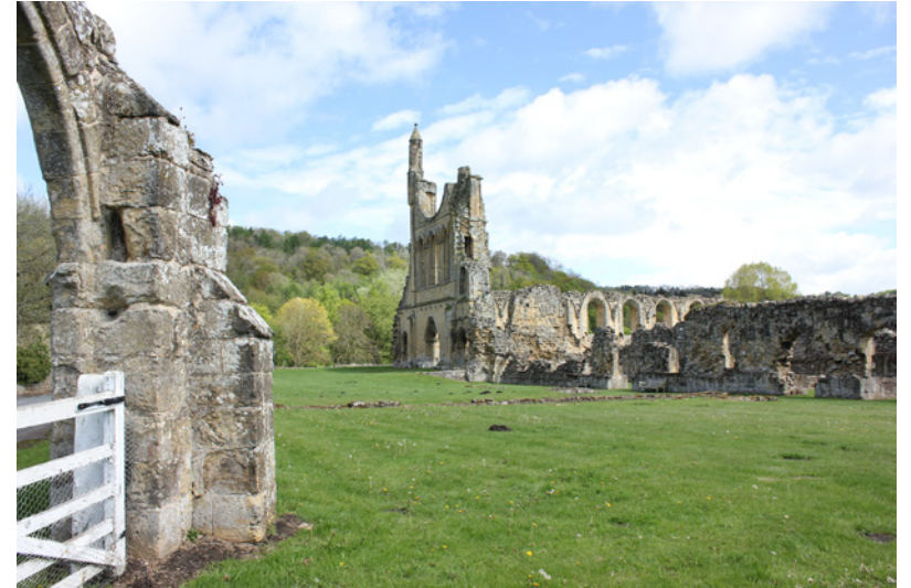
The west front looking north-east from the south of the site.
