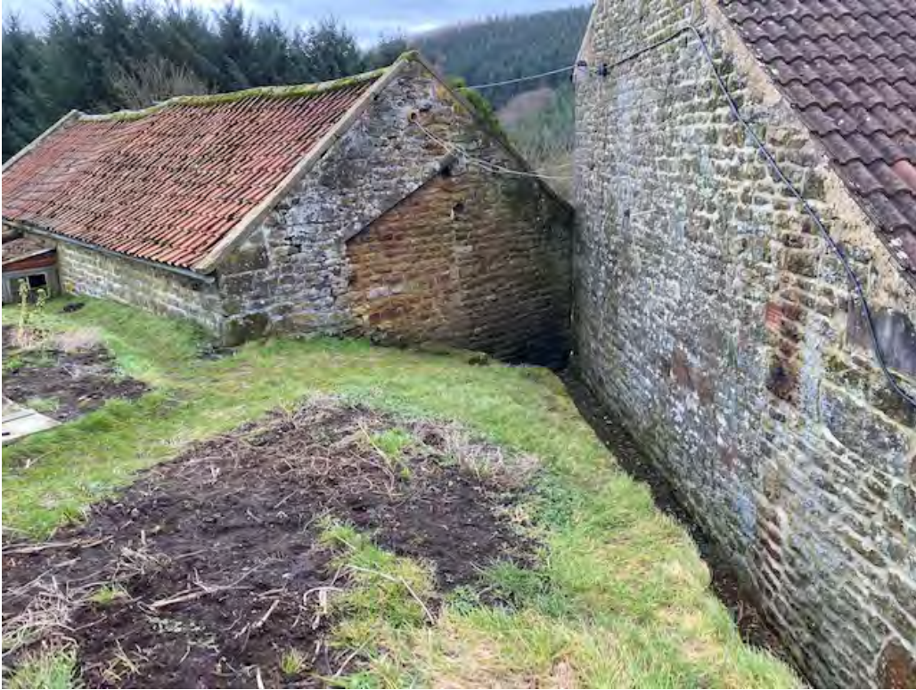
View higher up showing where proposed link will be constructed.
