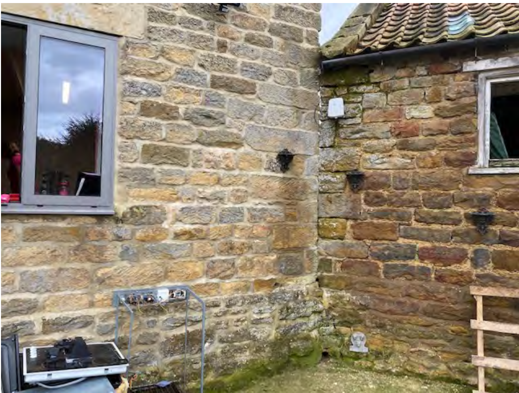
View where main dwelling meets existing stable block at the front
