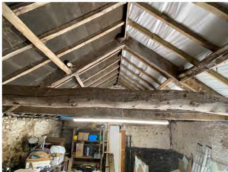
Plate 3 – internal roof void.
