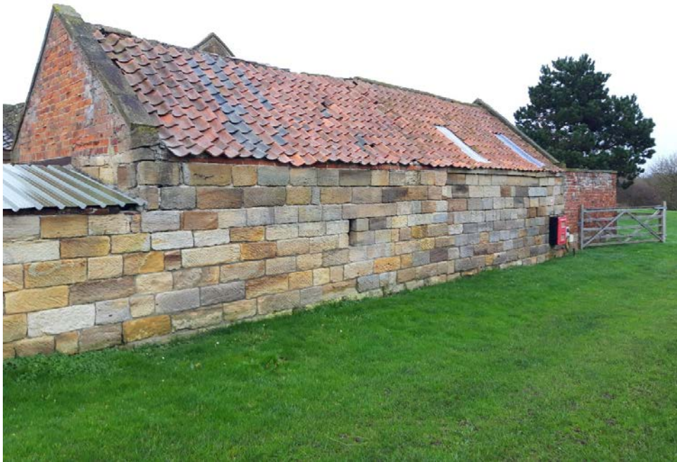
This photograph shows the south elevation of Building C.
