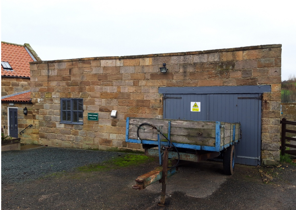
This photograph shows the north elevation of Building B.
