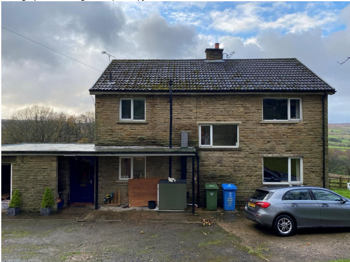
Photograph 2 – View of front of house from access drive
