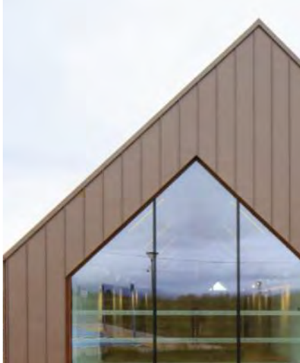
Metal trims to match window frames to timber buildings, to match standing seam to metal elevations
