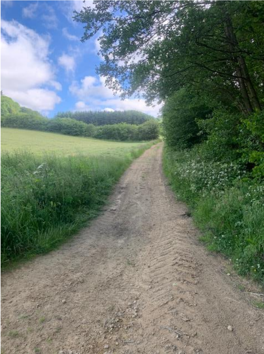
Picture indicative of the tracks that have been levelled and repaired only - Tracks 4,5,6,7 & 8
