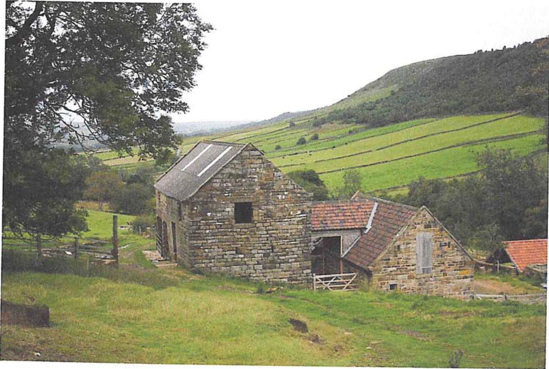
The buildings today From the South West
