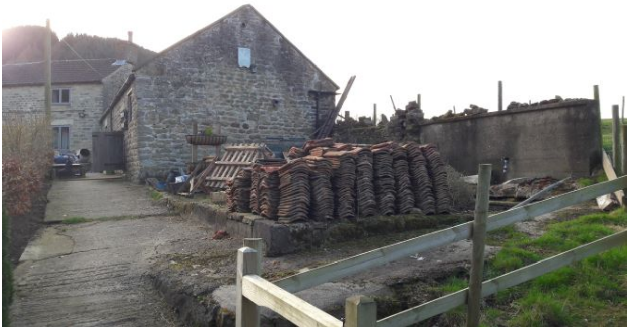
Gable elevation of stable showing previously developed site now used as outdoor storage area (pantiles, timber, materials etc.). This area is the site of the proposed glasshouse.
