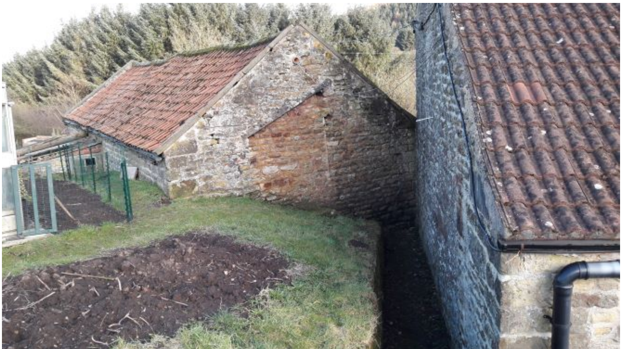
Rear of the stable building showing higher ground and triangular-shaped gap between the house gable and stable gable. This is the site of the proposed link structure.
