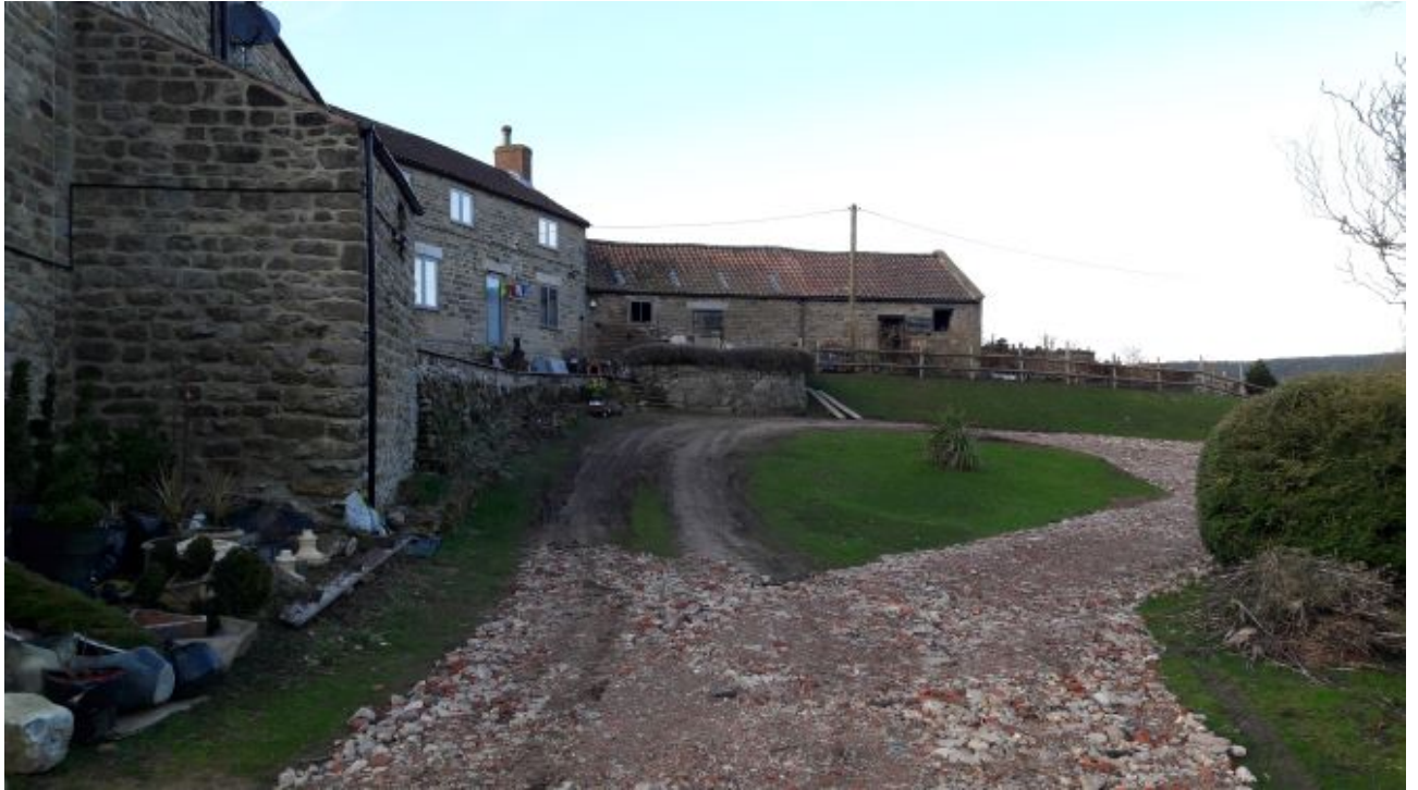
Approach to property showing main house to the left and the stable building to be converted in the centre of the picture. The stable is a single storey stone under pantile building comprising two large stables; each with a stable door and square eaves level window arranged as a mirror image.
