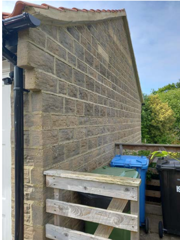
East elevation of the detached garage at 19 Hermitage Way, Sleights.
