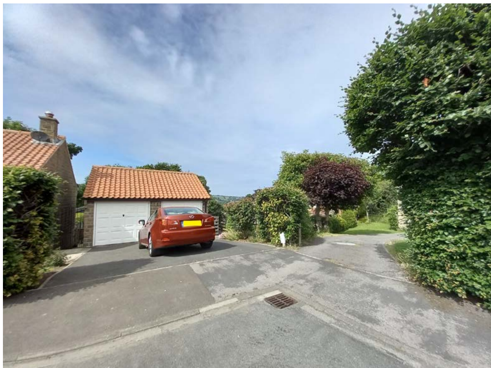
Front elevation of the detached garage at 19 Hermitage Way, Sleights.
