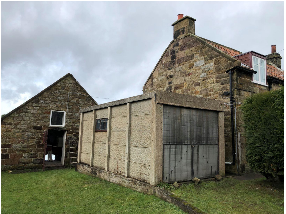
Photograph 1 Side Elevation, Pre-Cast Garage
