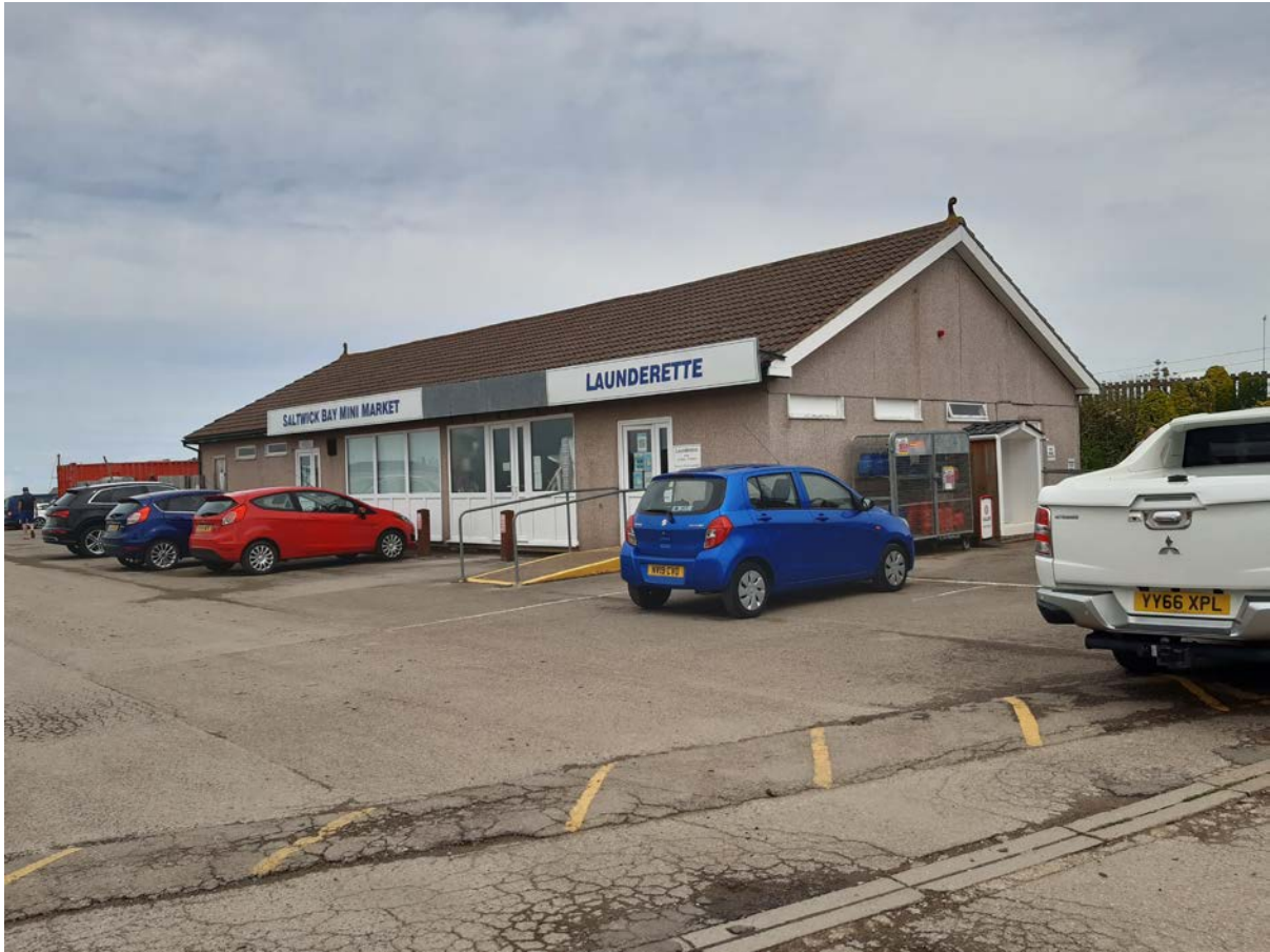
Front and side elevation of building for renovation
