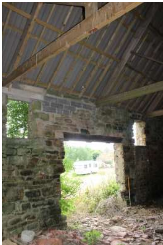
Plate 150: Internal view SW of the third compartment of Building No.4
