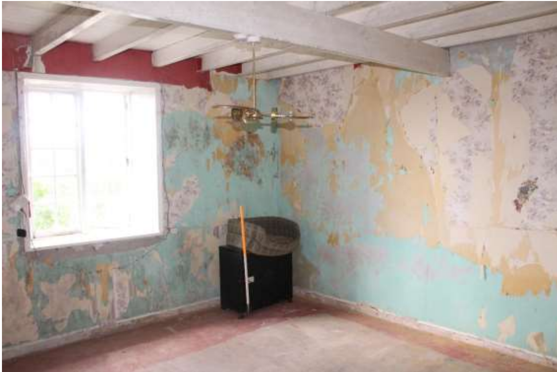
Plate 41: internal view SE within ground sitting room – Building No. 1
