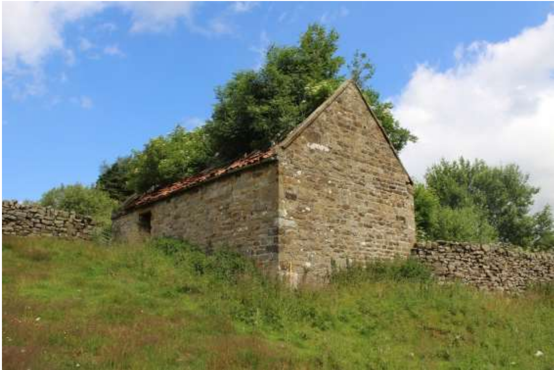
Plate 113: External oblique view of W and S-facing elevations of Building No. 3
