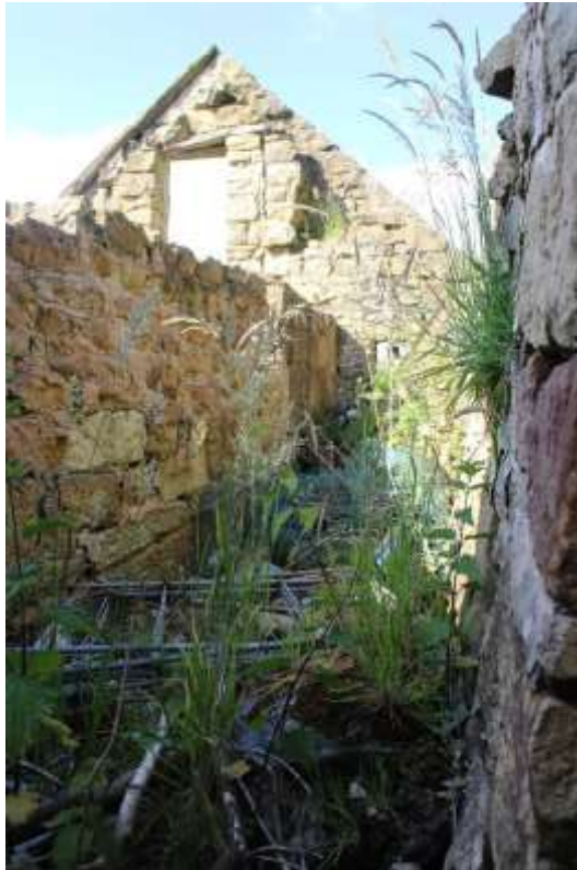
Plate 57 internal view SW of pigsty rear corridor – Building No. 1
