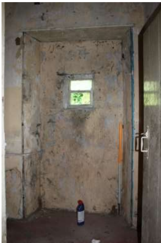
Plate 32: internal view NNW within ground toilet room, showing sash window within blocked up doorway – Building No. 1
