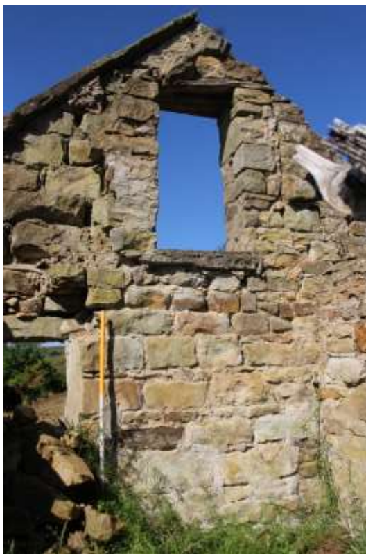
Plate 54: internal view W of pigstyes W partition showing upper floor entrance— Building No. 1
