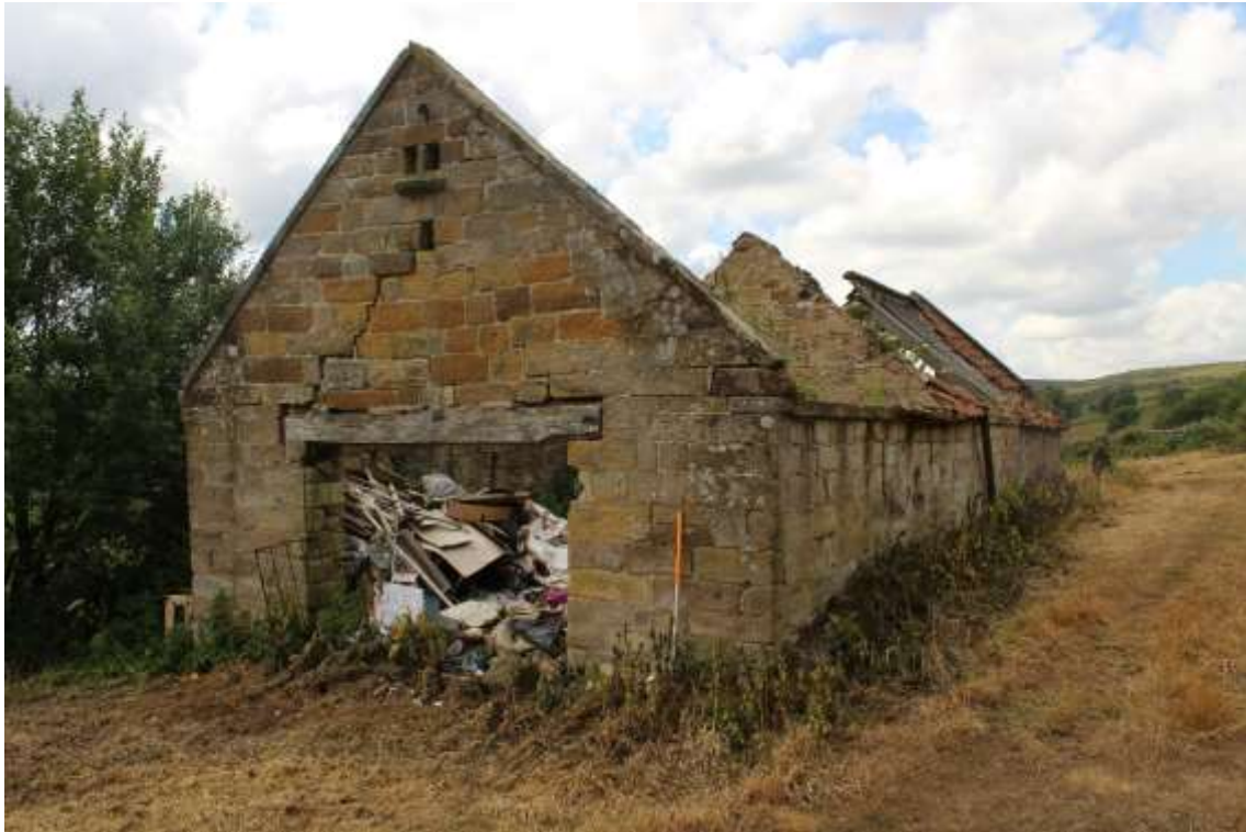
Plate 99: Exterior view SW of the N and E elevations of Building No. 2
