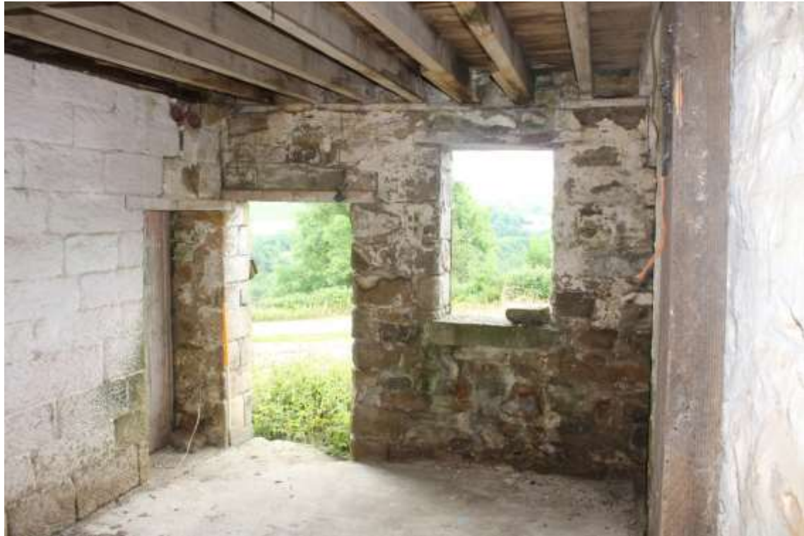
Plate 139: Internal view S of the second compartment of Building No.4
