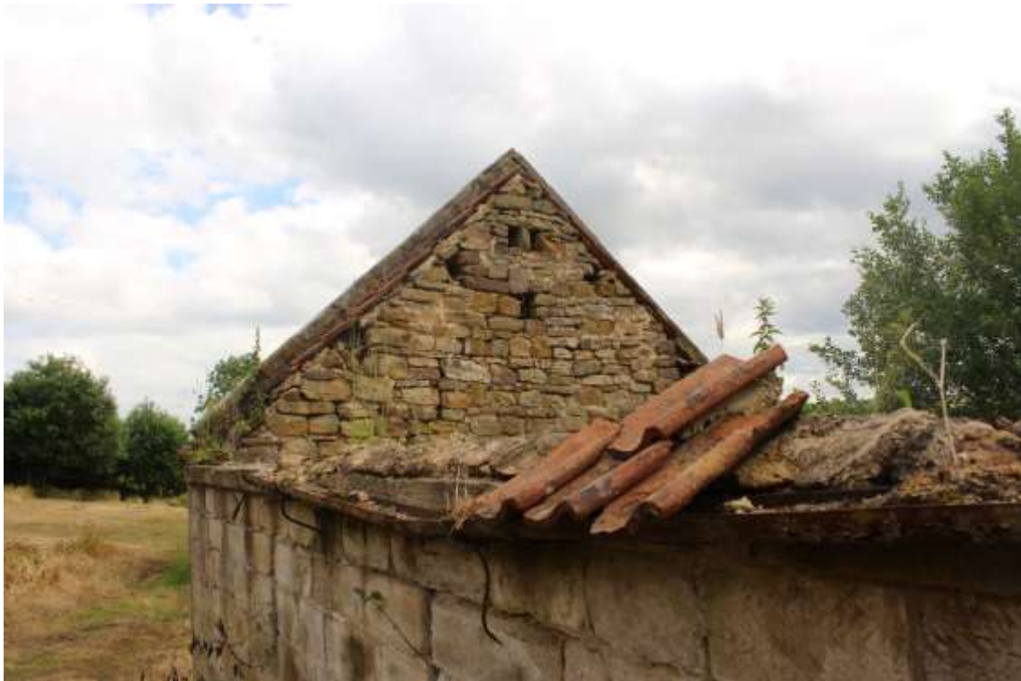
Plate 102: Close up view of interior E gable of Building No. 2
