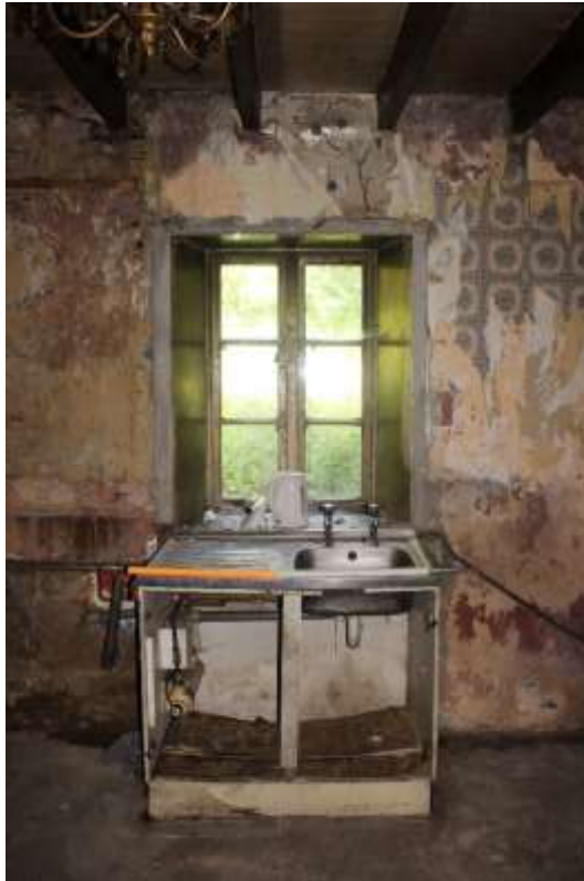
Plate 29: internal view NNW within ground floor kitchen showing casement window – Building No. 1
