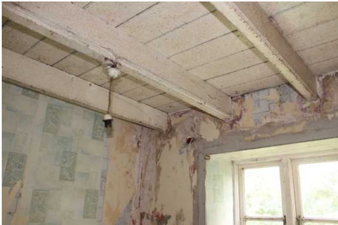
Plate 76: Internal view NNW of 1 st floor bathroom showing ceiling – Building No.1
