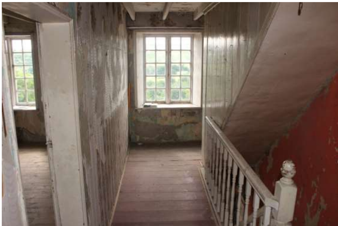
Plate 60: Internal view SSE of 1 st floor central hall way – Building No.1
