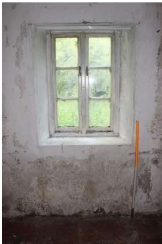
Plate 36: internal view NNW within ground floor storage room showing casement window within N wall— Building No. 1
