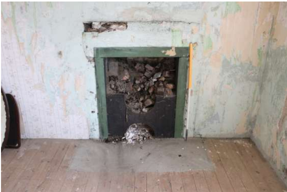
Plate 86: Internal view ENE of 1 st floor fourth bedroom fireplace – Building No.1
