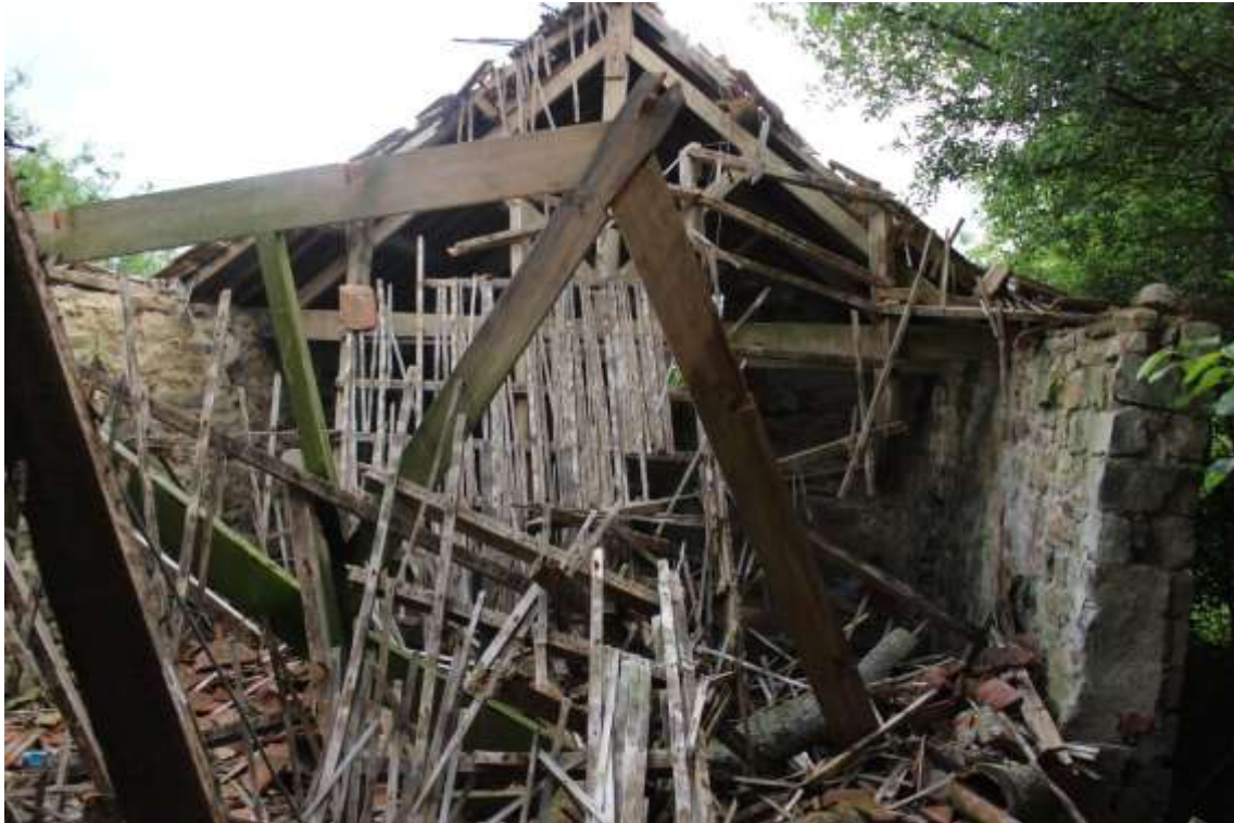
Plate 145: Internal view E from the third compartment into the fourth compartment of Building No.4
