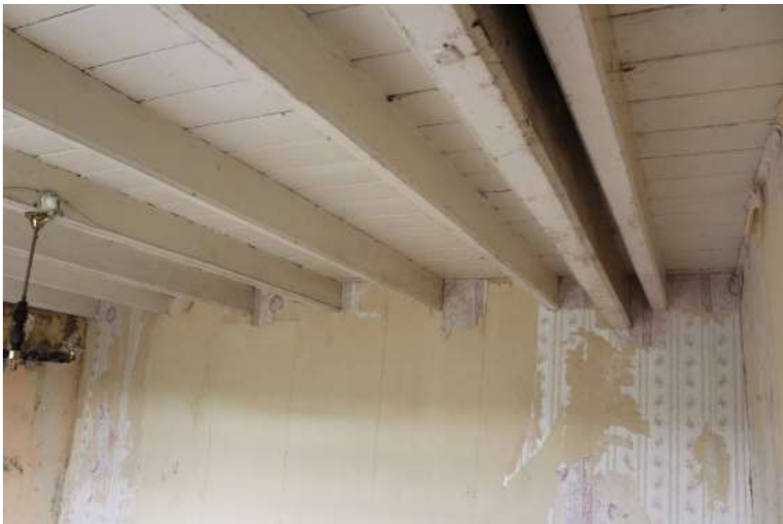
Plate 68: Internal view NW of 1 st floor bedroom showing ceiling – Building No.1
