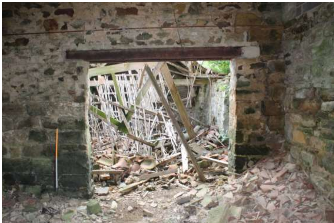
Plate 144: Internal view E of the third compartment of Building No.4
