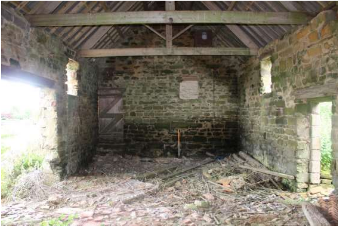
Plate 147: Internal view W of the third compartment of Building No.4
