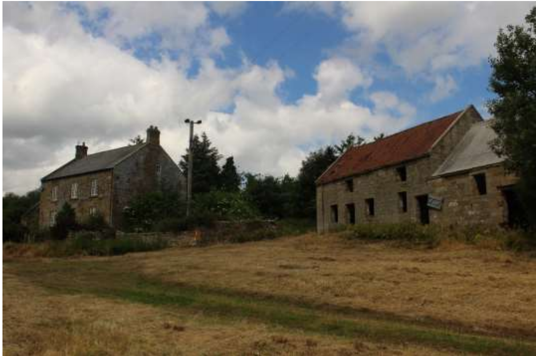
Plate 1: View NW showing farmhouse (Building No. 1 - left) and combination barn (Building No. 4 - right)
