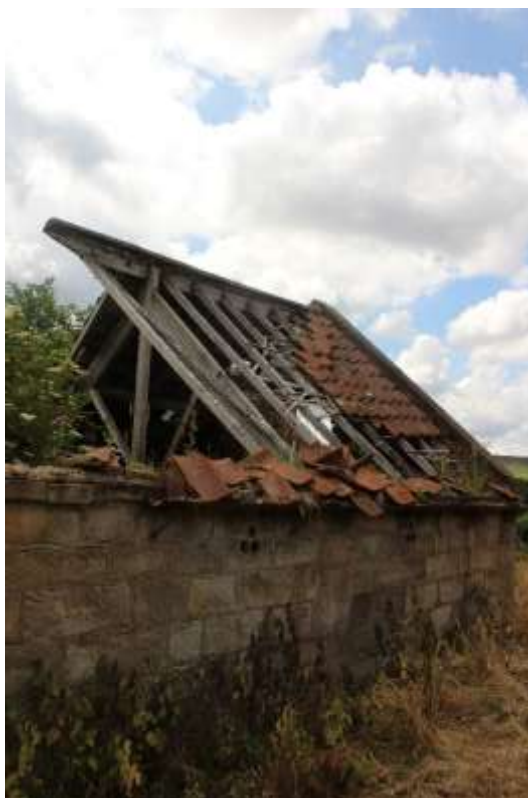
Plate 104: Oblique view SSW of N-facing elevation of Building No. 2
