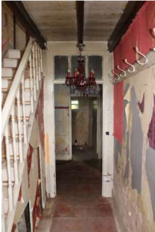
Plate 13: Internal view NNW along the ground floor central hall of the farmhouse – Building No. 1
