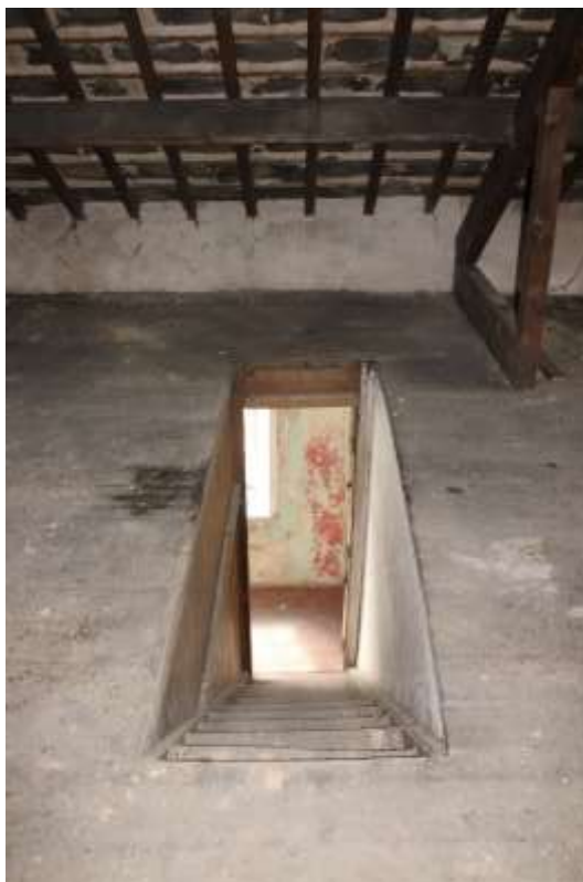
Plate 88: Internal view SSE of stair case leading to the 1 st floor from the attic/roof space – Building No.1
