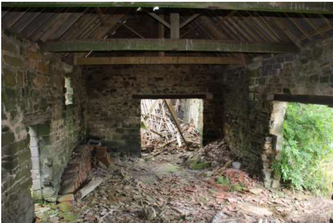
Plate 142: Internal view E of the third compartment of Building No.4
