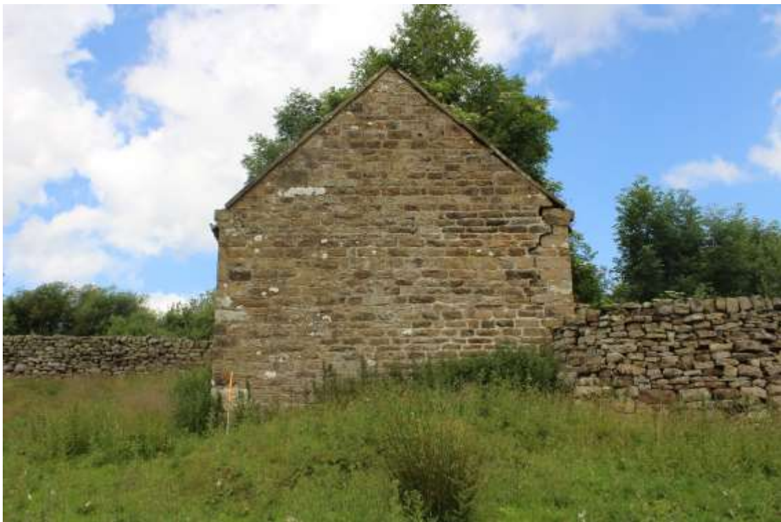
Plate 114: External view NNW of S-facing gable end of Building No.3
