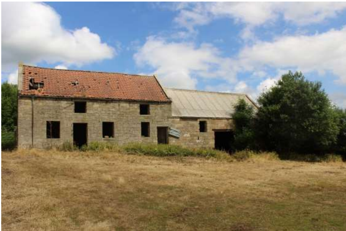
Plate 118: External view N of principal S-facing elevation of Building No. 4
