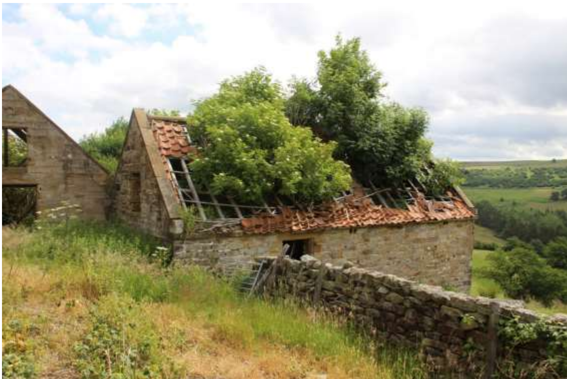
Plate 110: Oblique view ESE of N and W-facing elevation of Building No.3
