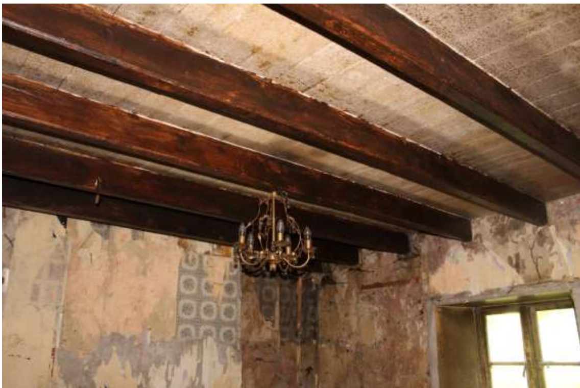
Plate 30: internal view WNW within ground floor kitchen showing ceiling – Building No. 1
