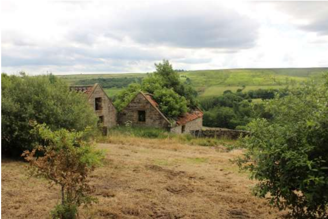
Plate 109: Oblique view ESE of Buildings No. 2 & 3
