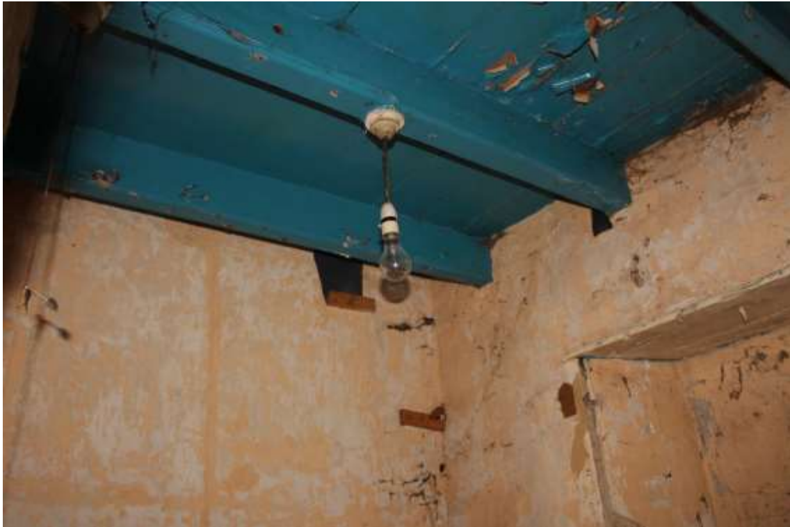
Plate 33: internal view WNW within ground toilet room showing ceiling— Building No. 1
