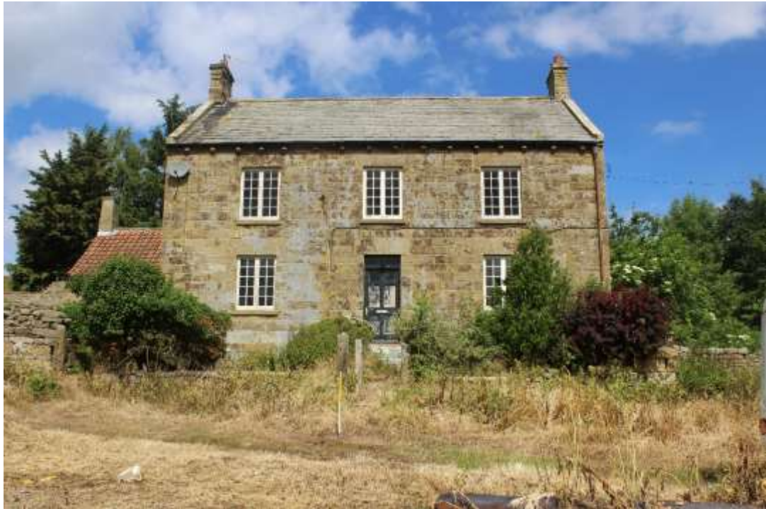
Plate 3: View NNW showing S elevation of the farm house Building No.1
