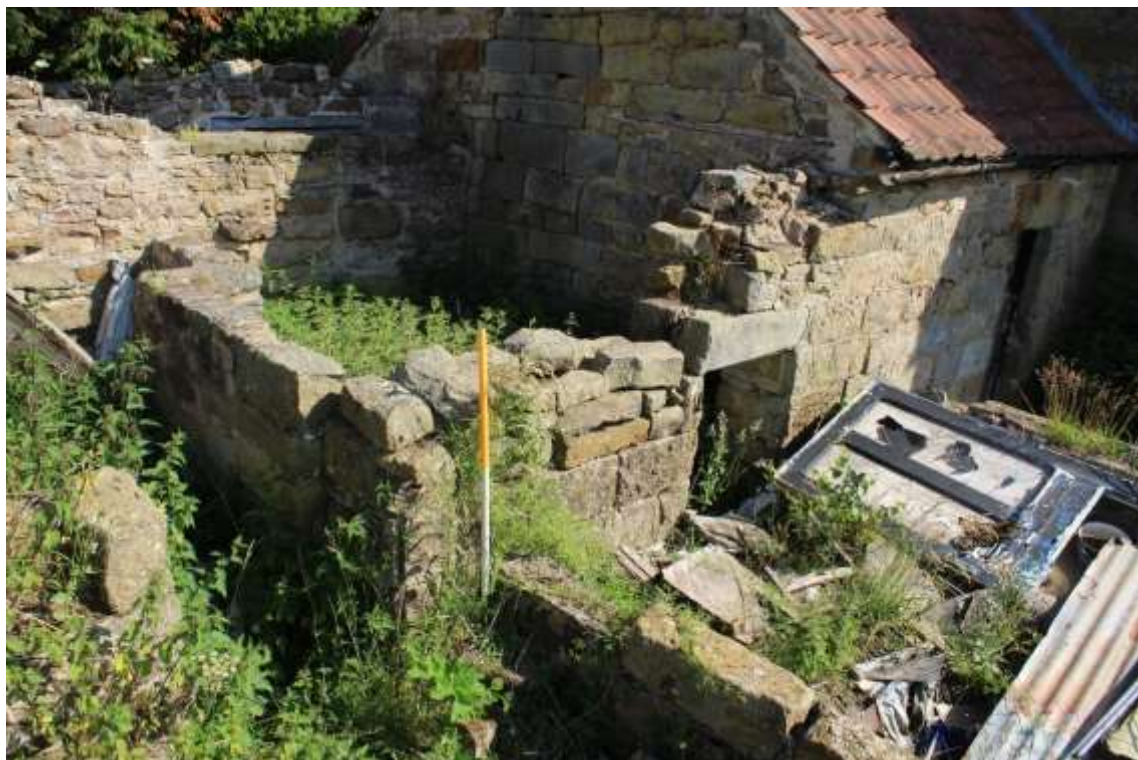
Plate 58: internal view NNE of pigsties E partition – showing half height door opening onto yard Building No. 1
