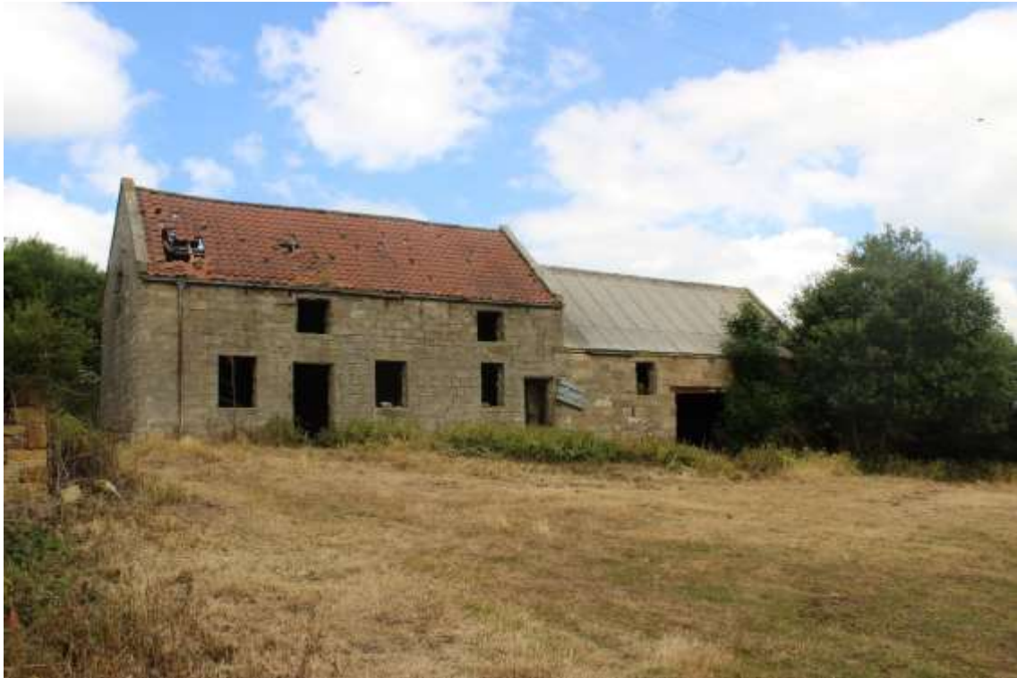
Plate 117: External oblique view NNE of the principal S facing elevation and W-facing elevation of Building No.4
