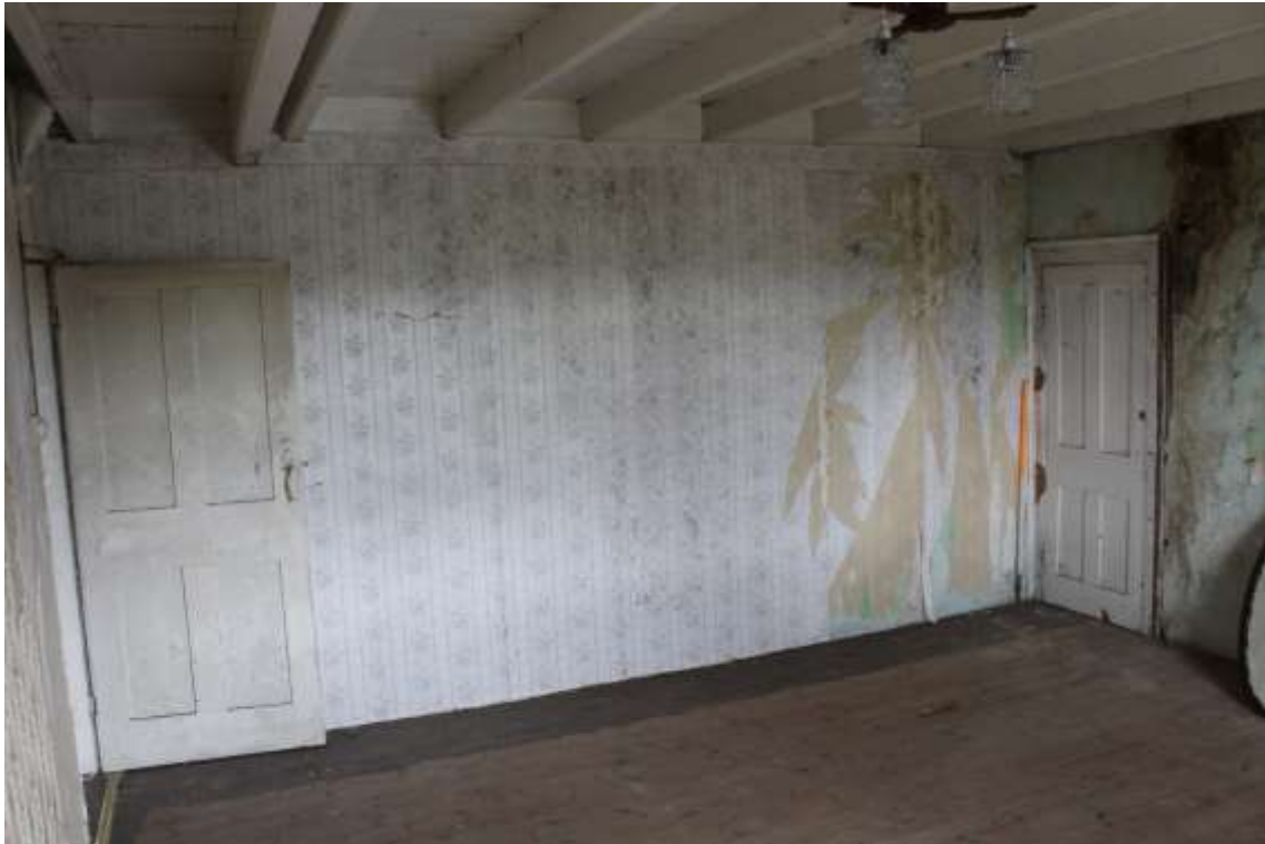
Plate 83: Internal view NNE of 1 st floor fourth bedroom showing locked storage alcove – Building No.1
