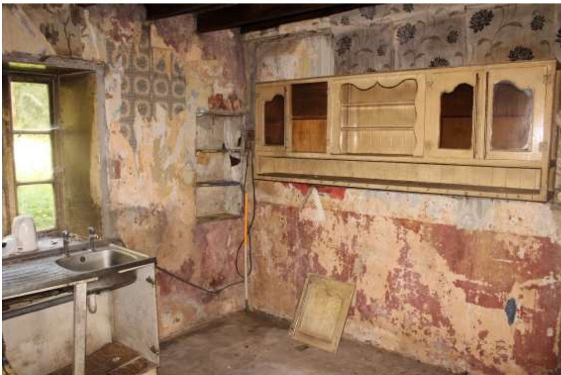
Plate 28: internal view NNE within ground floor kitchen – Building No. 1
