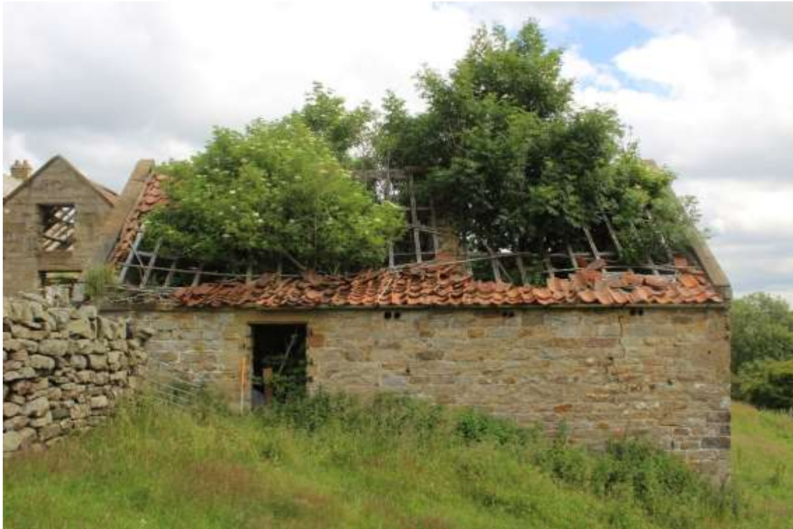
Plate 111: Exterior view WSW of the E elevation of Building No. 2
