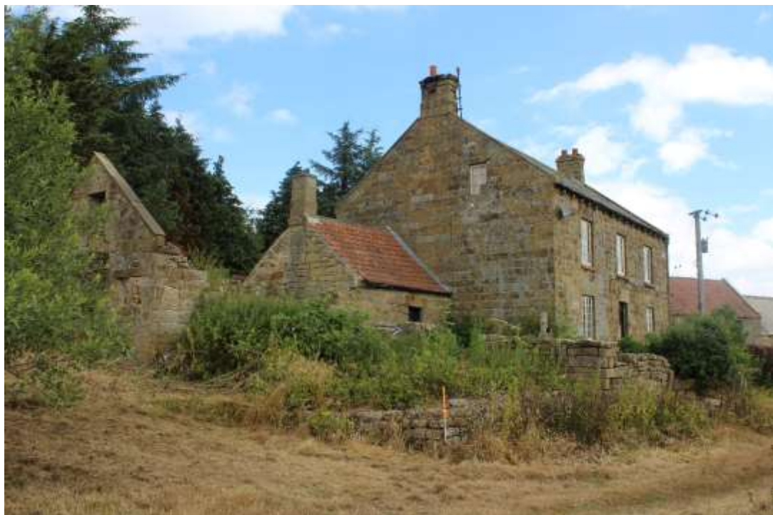
Plate 4: View NE showing S facing elevation of the farmhouse Building No.1, with derelict pigsty (foreground) and outbuilding (middle foreground)
