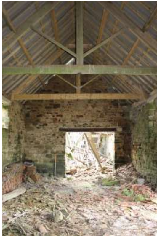
Plate 143: Internal view E of the third compartment of Building No.4
