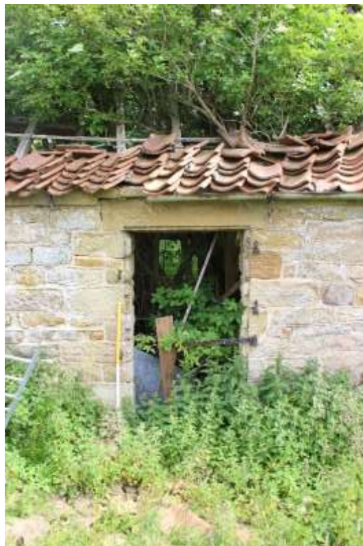
Plate 112: Close up external view ENE of stable door with W-facing elevation of Building No.3
