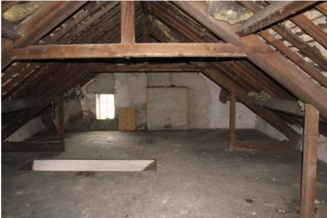
Plate 91: Internal view WSW of attic/roof space – Building No.1
