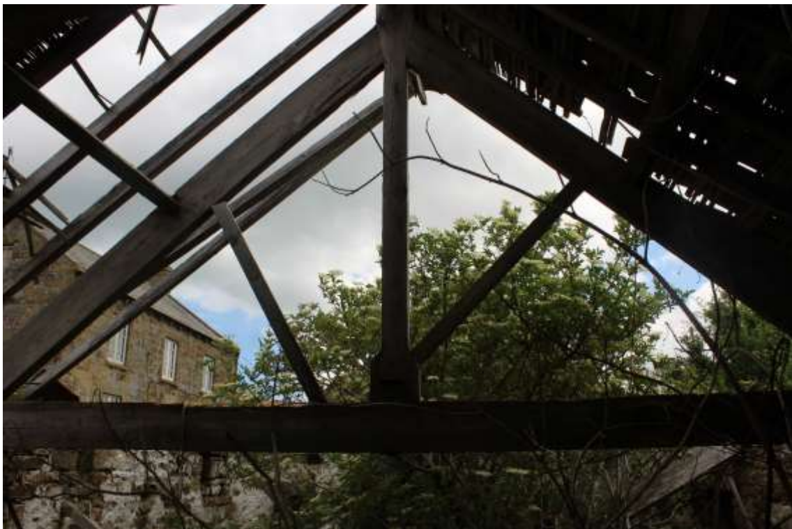
Plate 108: Internal view ENE of surviving king post truss with W compartment of Building No. 2
