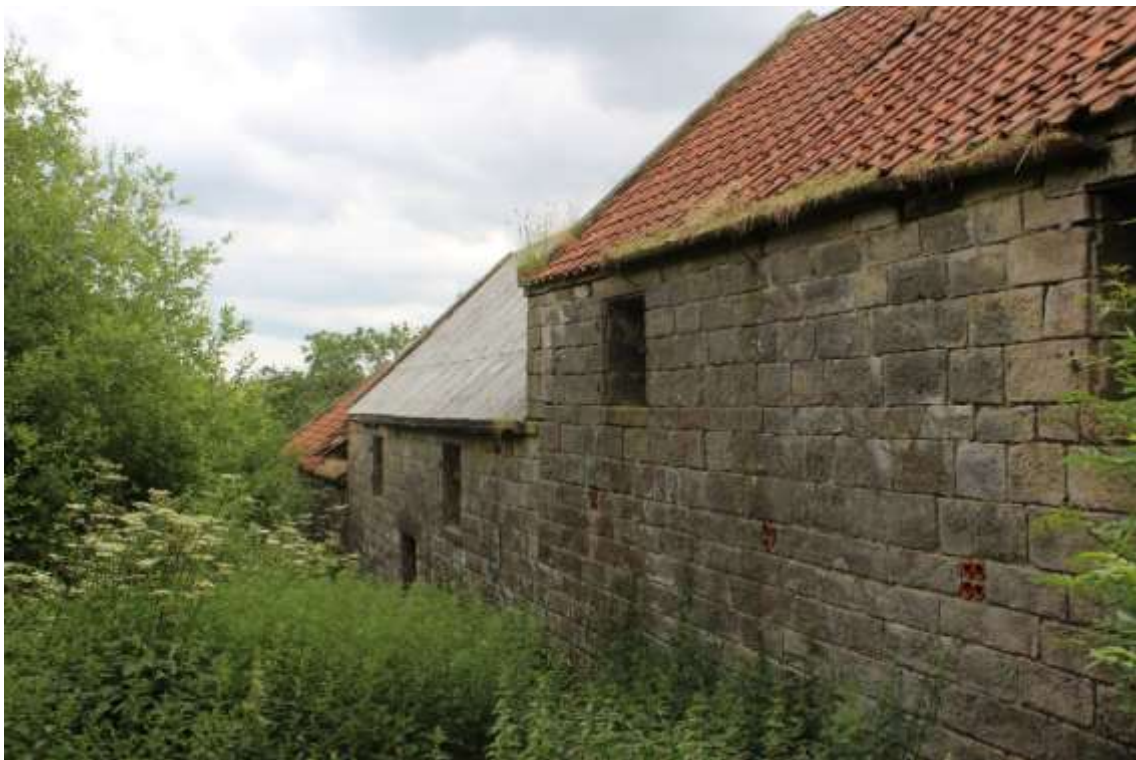
Plate 124: Oblique external view ESE of N-facing elevation of Building No.4
