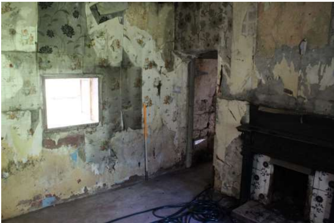
Plate 26: internal view SSW within ground floor kitchen – Building No. 1
