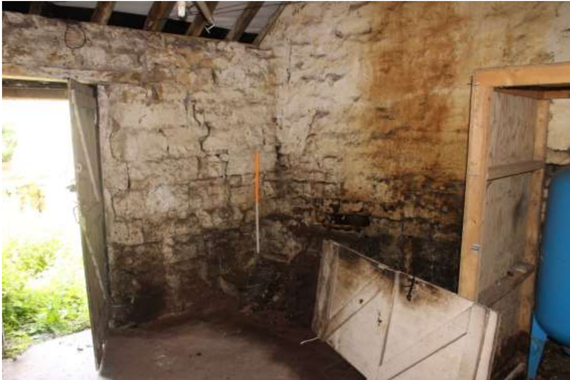
Plate 45: internal view SW within ground floor outhouse showing the remains of a corner stove– Building No. 1
