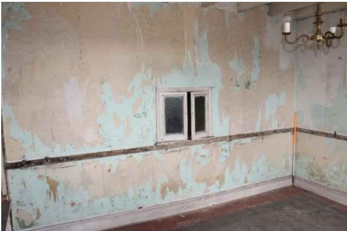
Plate 22: internal view ESE within ground floor living room showing service hatch through to the kitchen – Building No. 1
