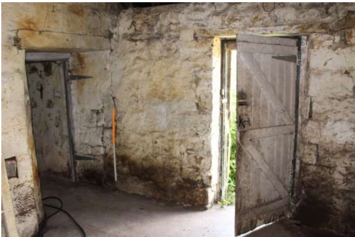
Plate 46: internal view SE within ground floor outhouse – Building No. 1
