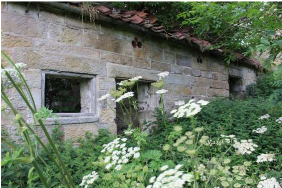
Plate 116: External oblique view of E-facing elevation of Building No.3
