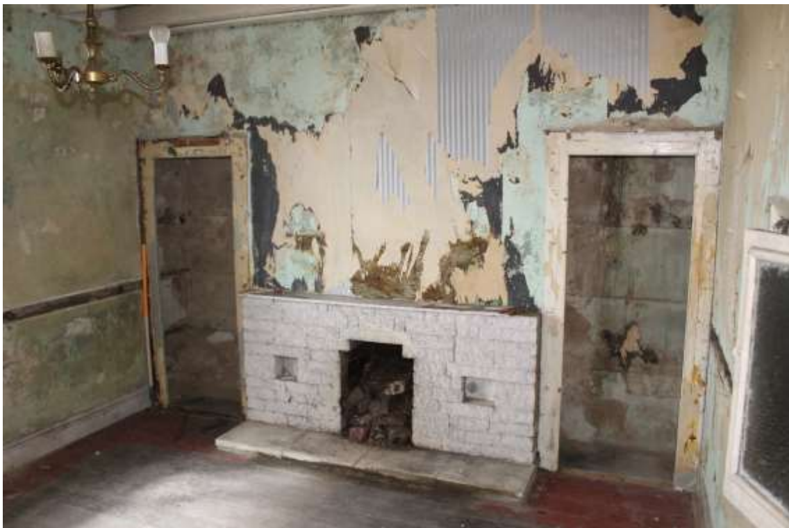
Plate 20: Internal view W within ground floor living room showing central fireplace and built in cupboards – Building No. 1
