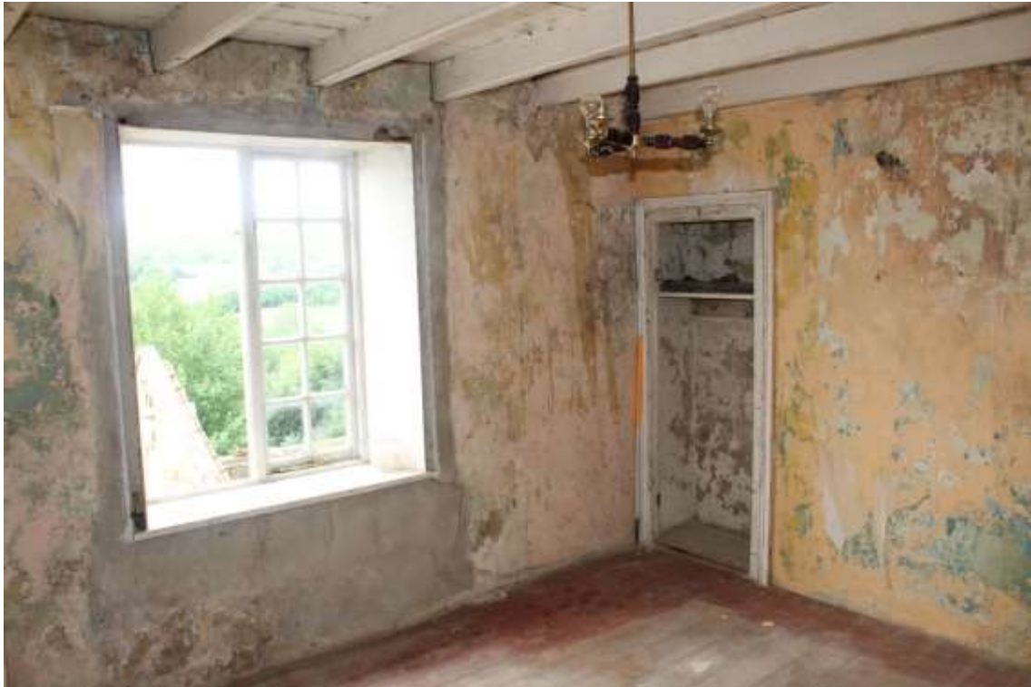
Plate 65: Internal view SW of 1 st floor bedroom showing two light casement window in N wall– Building No.1
