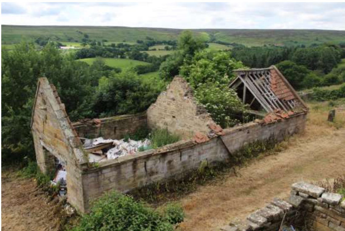
Plate 96: Exterior view SSW of derelict barn - Building No. 2
