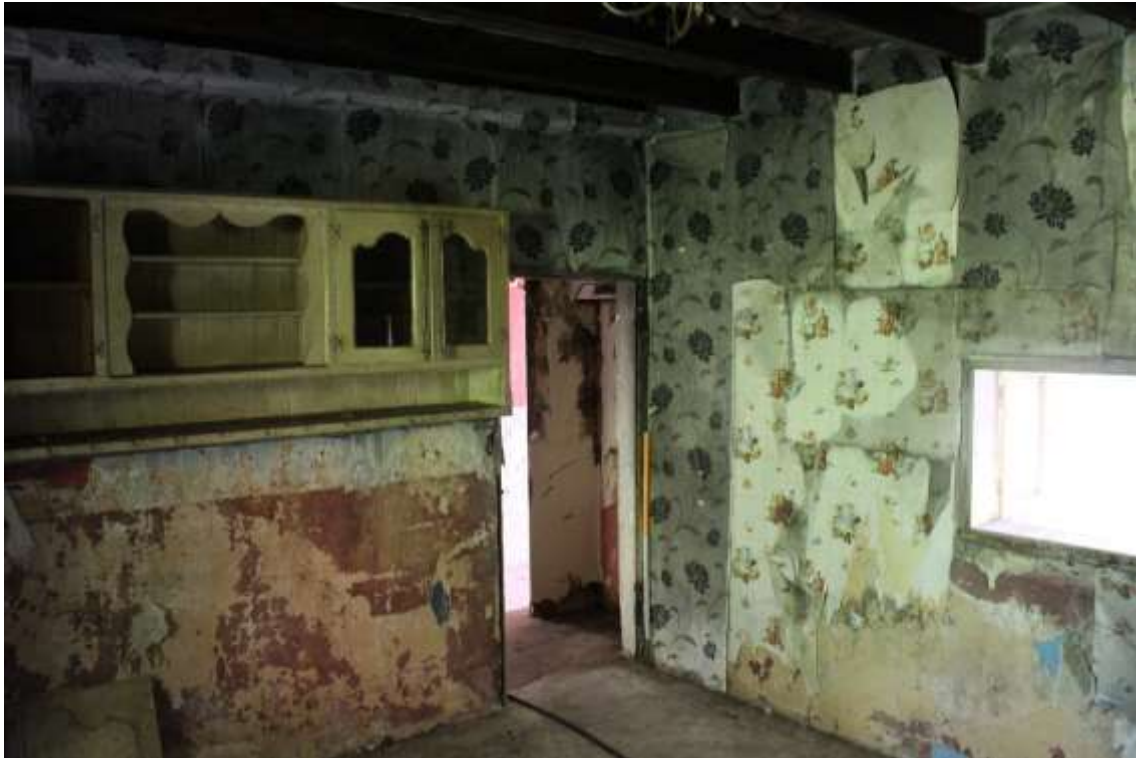
Plate 27: internal view ESE within ground floor kitchen – Building No. 1
