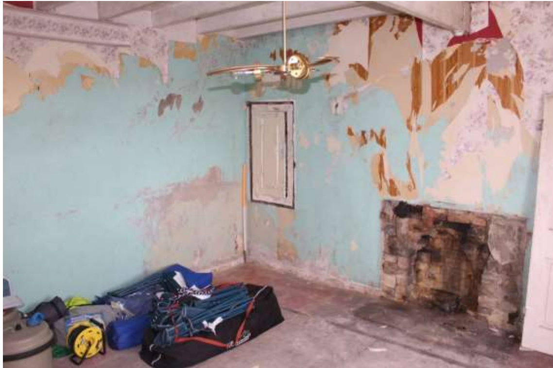
Plate 39: internal view SE within ground sitting room – Building No. 1
