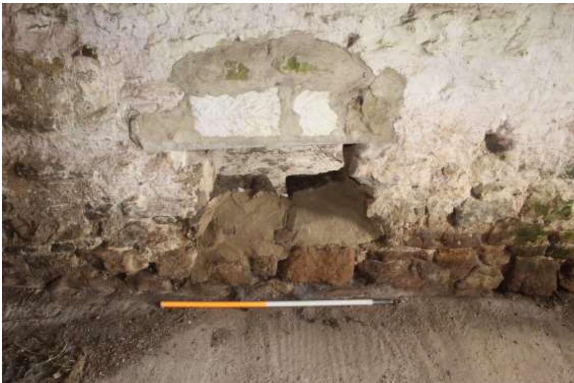
Plate 134: Internal view E of hole in E wall within the first compartment of Building No.4
