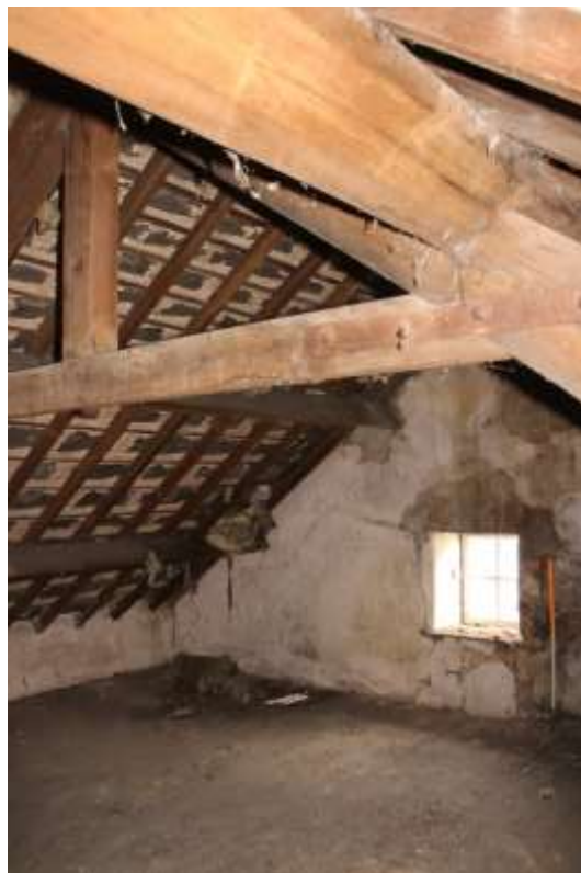
Plate 94: Internal oblique view SSW of attic/roof space showing single light casement window – Building No.1
