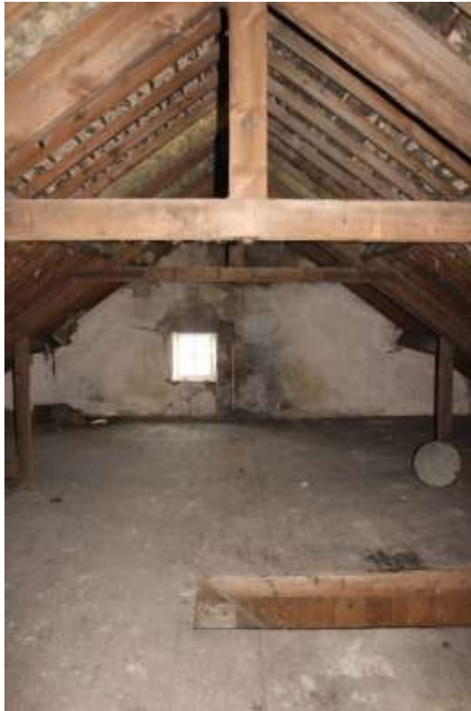
Plate 89: Internal view ENE of attic/roof space – Building No.1
