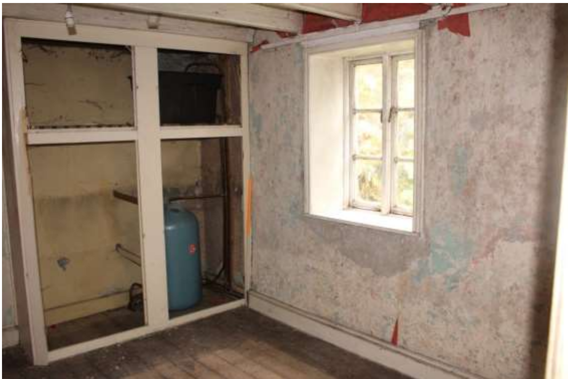
Plate 72: Internal view SW of 1 st floor second bedroom showing two light casement window within N wall – Building No.1
