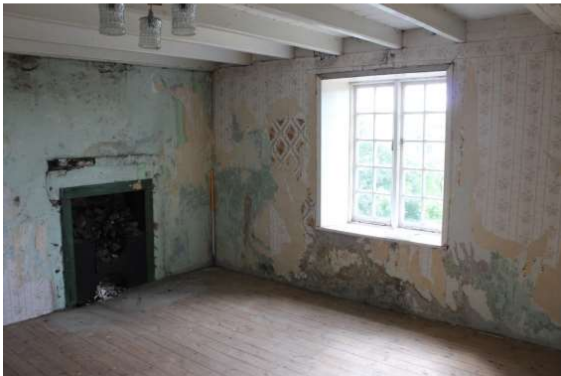
Plate 81: Internal view SE of 1 st floor fourth bedroom showing two light casement window with S wall – Building No.1
