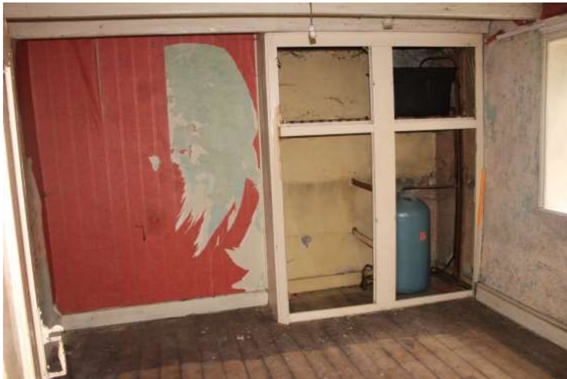
Plate 69: Internal view NW of 1 st floor second bedroom – Building No.1
