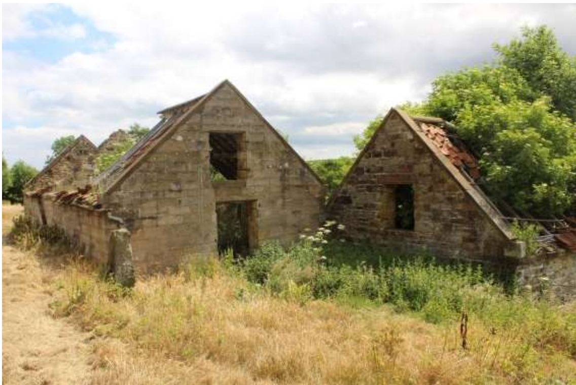
Plate 106: Oblique view ESE of Buildings No. 2 & 3
