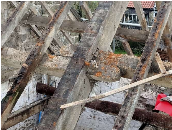
Purlin joint detail
