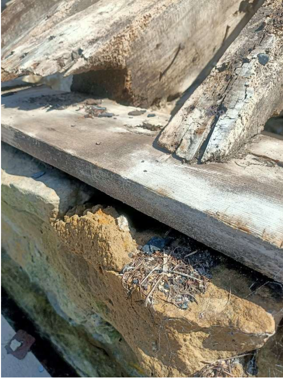
The picture shows the existing beam with the bird's mouth and existing wall plate
