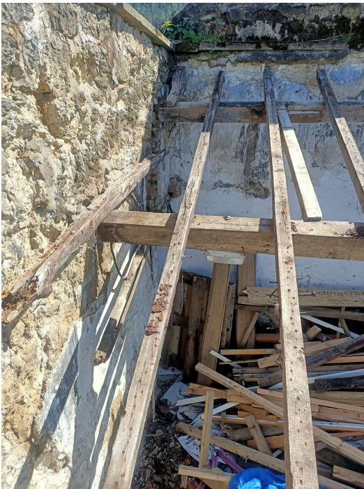
The picture shows the existing beam with the bird's mouth and existing wall plate
