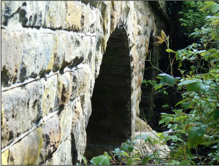
Figure 5: West side of bridge
