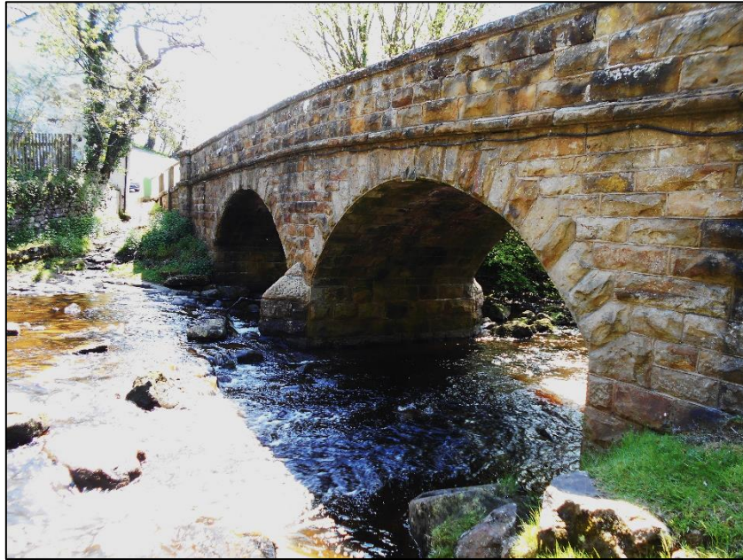
Figure 3: East side of bridge
