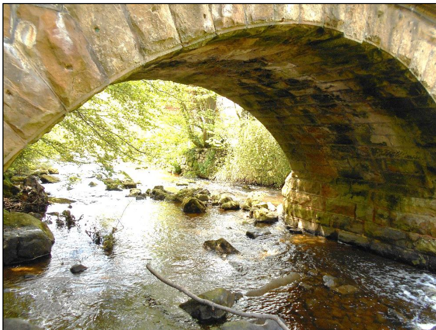
Figure 6: View towards west under south arch
