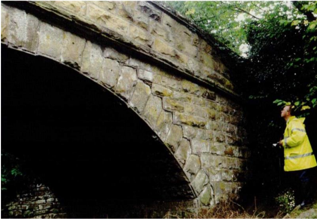
Downstream Elevation (SW Spandrel) – 1997
