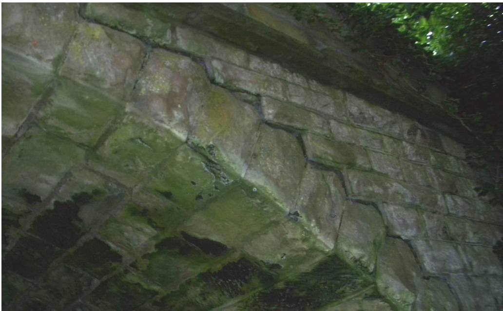
Downstream Elevation (SW Spandrel) - 2011
