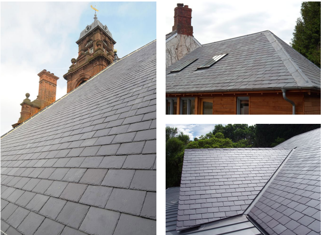
Fig. 2.1 Sample images of completed roofing projects in Welsh Slate Ltd. Penrhyn Heather Blue slate (images taken from: http://www.welshslate.com/gallery/?tag=penrhyn-heather-blue ).
