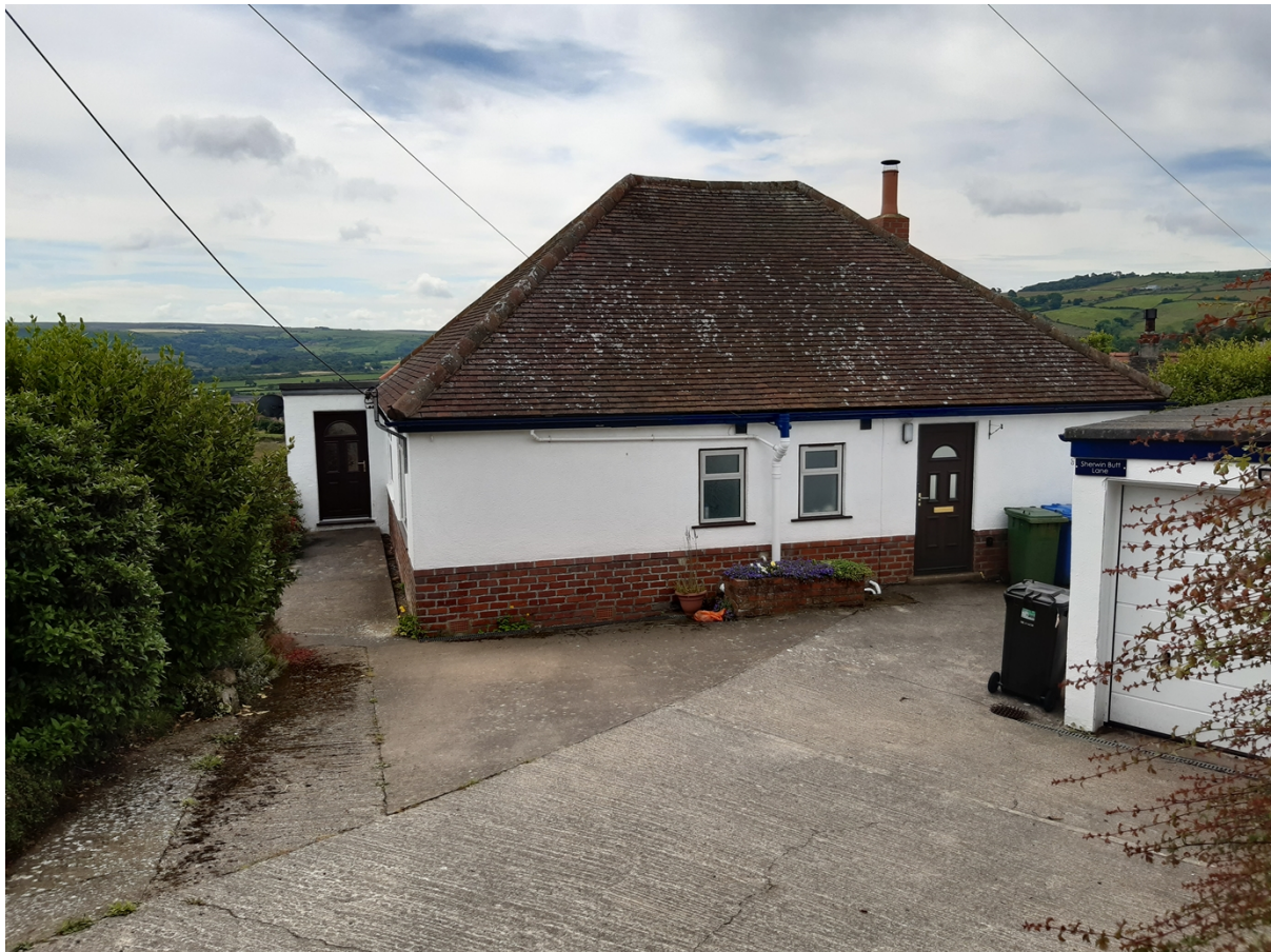
Rear elevation taken from Butt Lane – extension would be to the left side
