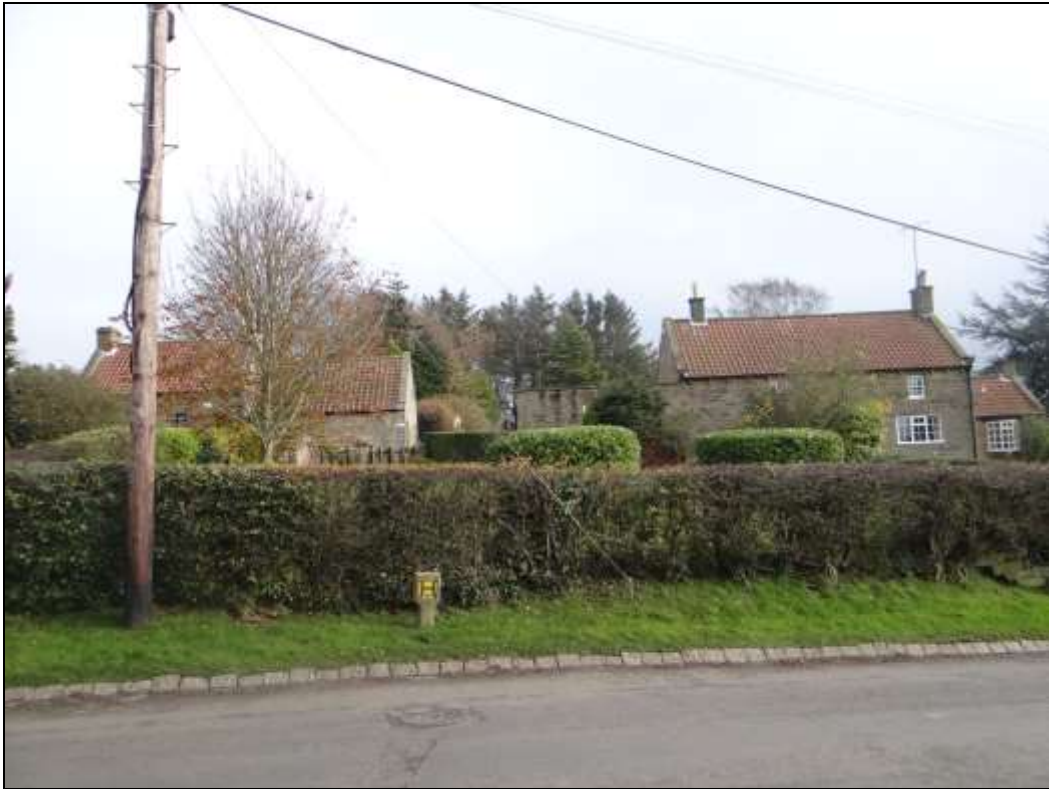
View of the cottage from the Highway (West elevations).
