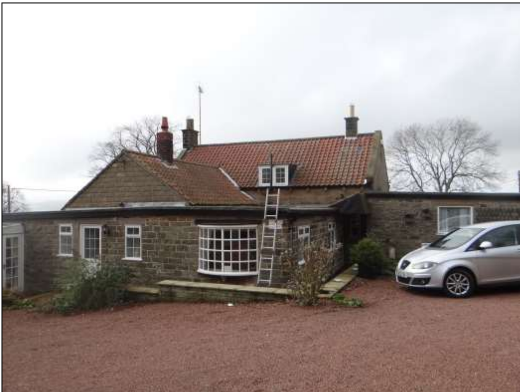
Rear view of the cottage (East elevations).
