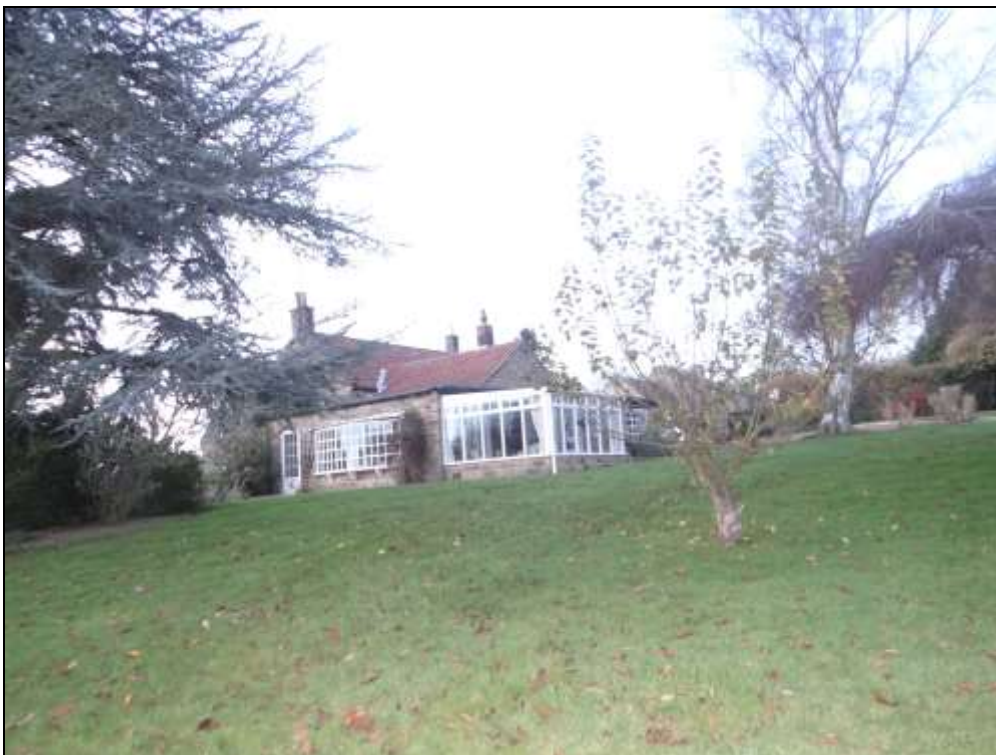
Rear view to the south east corner showing existing conservatory and the shallow/flat roofed extension.
