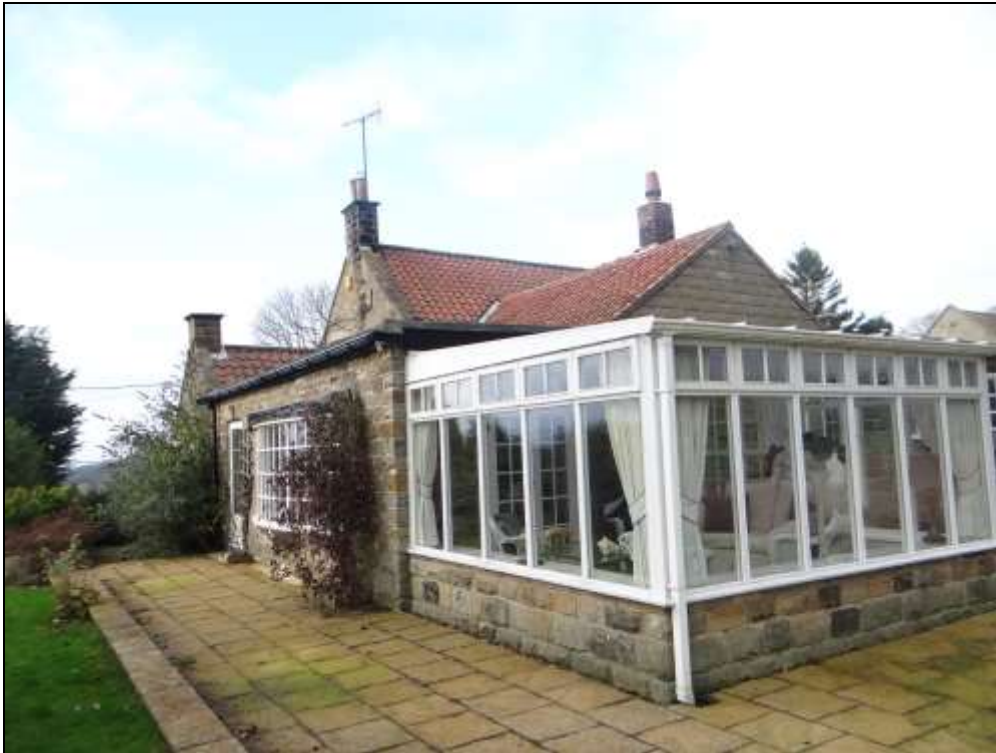
Rear view to the south east corner showing existing conservatory.
