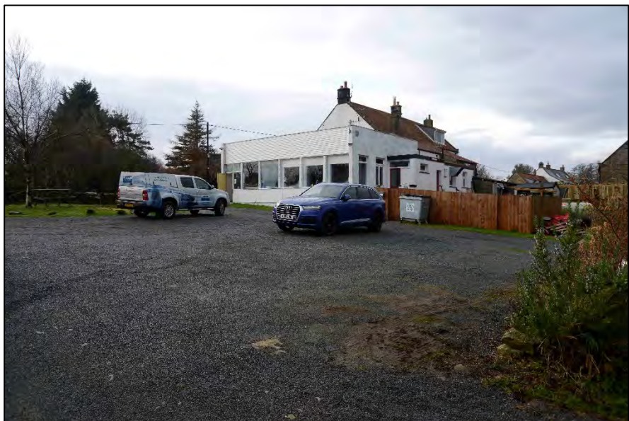
Appendix 2.6: View of the east elevation of Wilson Arms from the car park, looking west
