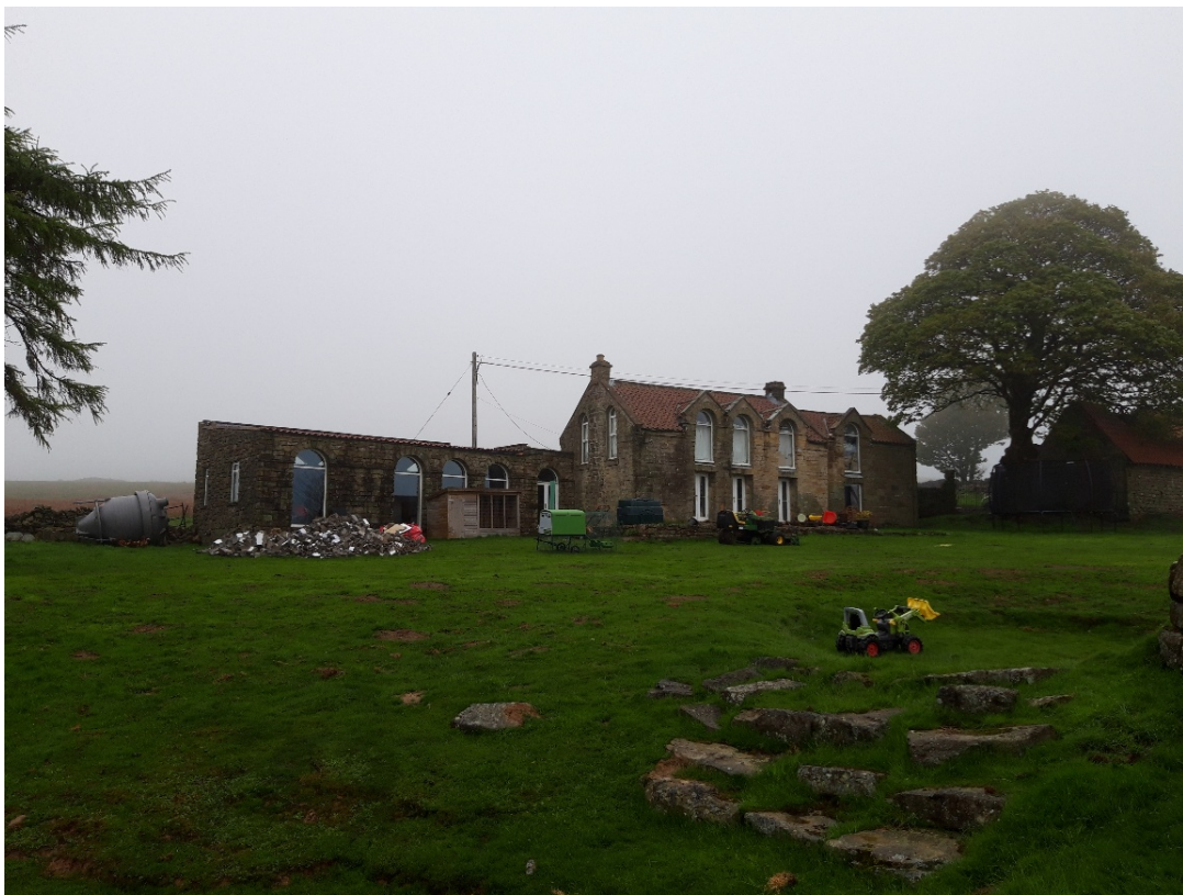
This photograph shows the southern elevation of the property.
