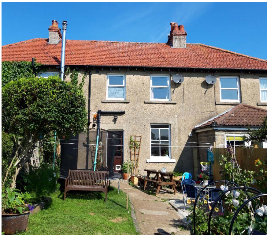
This photo shows the rear of 42 Iburndale Lane, where the proposed rear extension is to be constructed.
