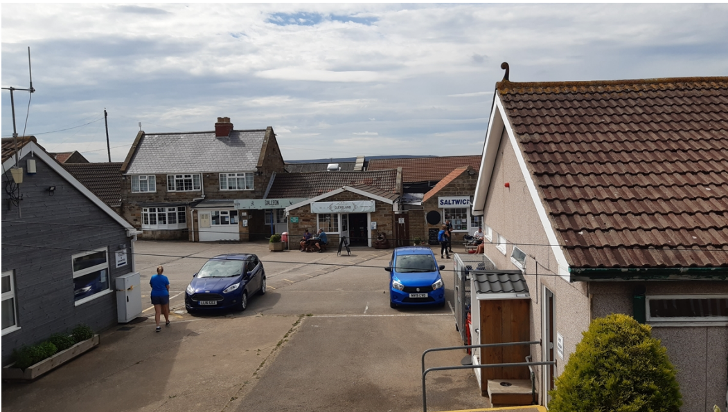
Photograph showing roof slopes for solar PV panels
