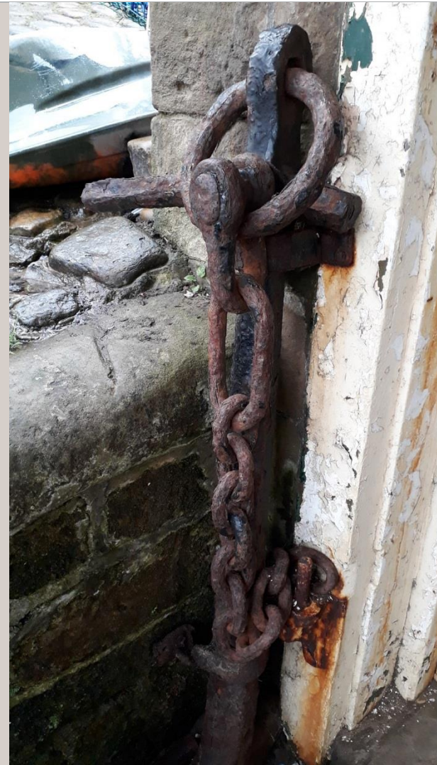
Figure 14: Anchor relocated to right side of canopy. A plaque above records that: "This old single fluke anchor was buried in the Dock and used as a "holdfast" during the launch and retrieval of Robin Hood's Bay's self-righting rowing lifeboats...The anchor was discovered in 1963 and it stands as a symbol of the ingenuity and bravery of generations of Robin's Hood's Bay volunteer lifeboat crews
