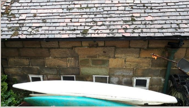
Figure 18: Detail of the second blocked historical window in the south elevation
