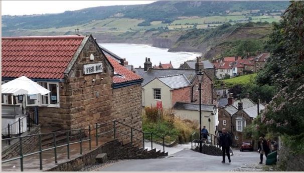
Figure 10: Approach to site down New Road. The application site is not visible in this view, which does however highlight the character and appearance of Robin Hood's bay
