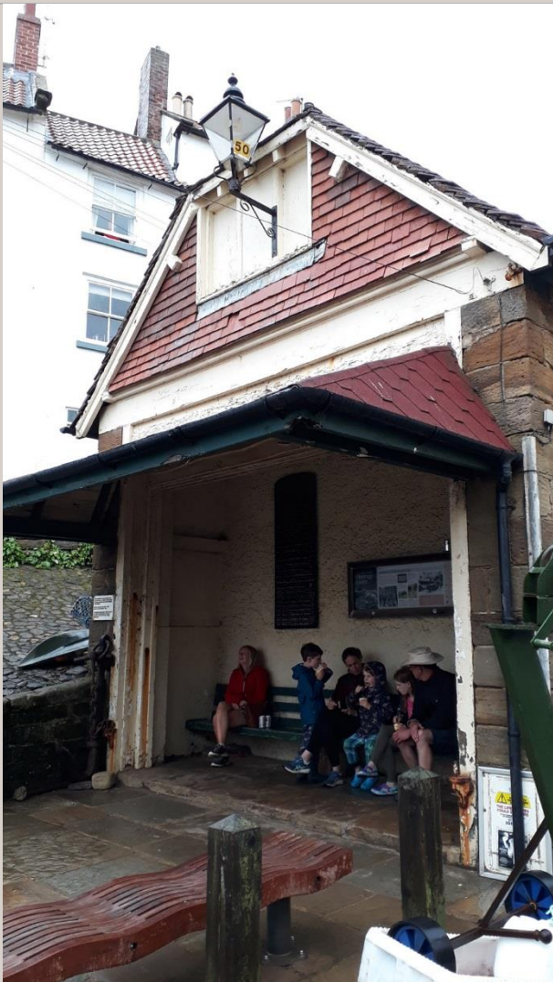
Figure 12: View to east gable facing sea with blocked window and inserted lamp with canopy below. The door surround to the original opening has been preserved and bench, floor, rear wall etc inserted in the c.1960s/1970s
