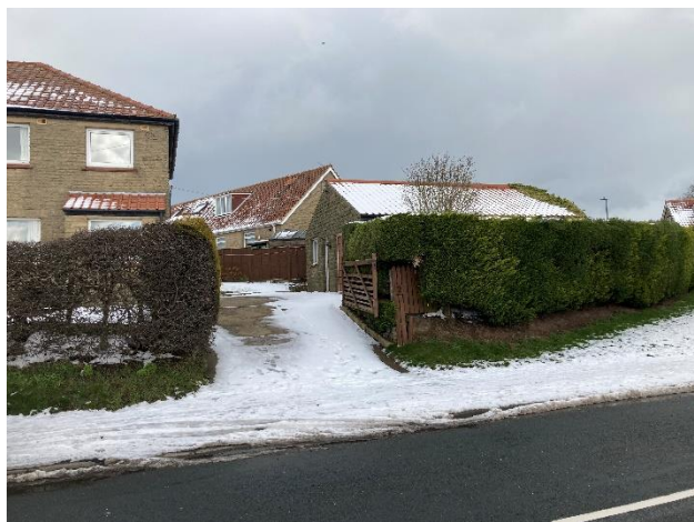
Fig 1. – House and outbuilding at 2 Prospect Field, Hawsker.
