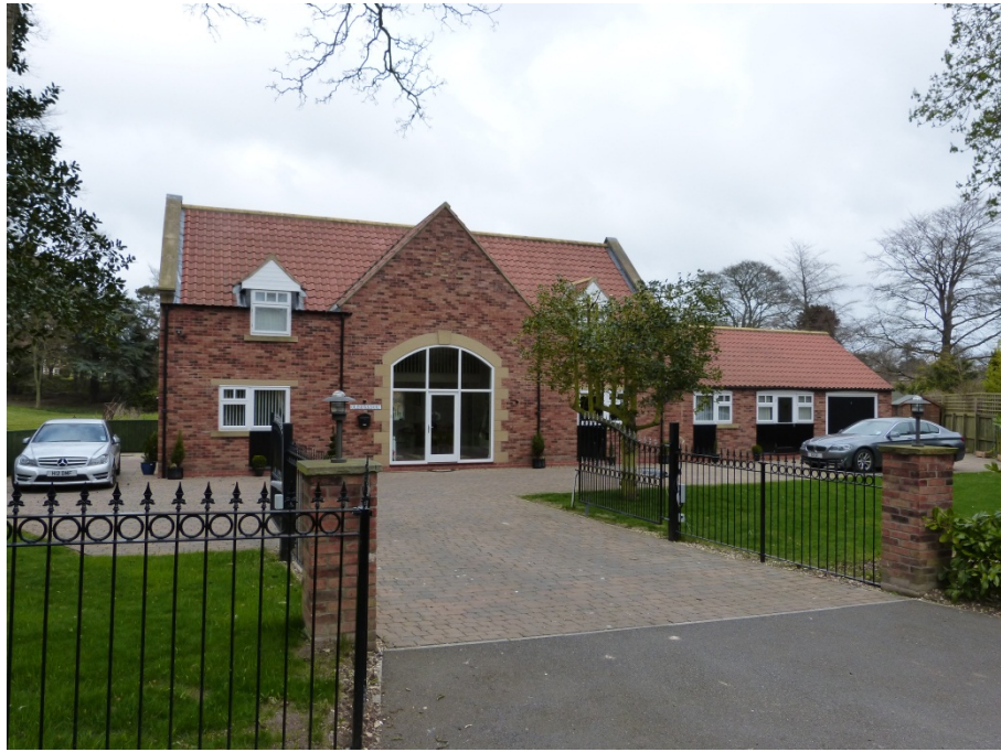
The just completed house 'B' next to the Lodge House
