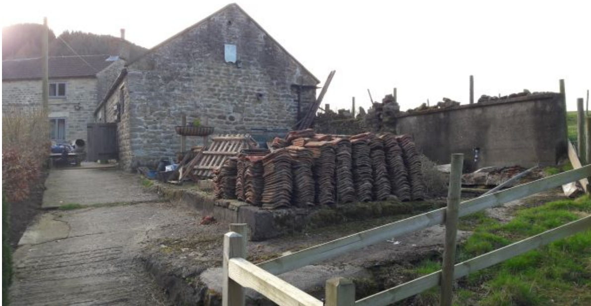
Gable elevation of stable showing previously developed site now used as outdoor storage area (pantiles, timber, materials etc.). This area is the site of the proposed glasshouse.
