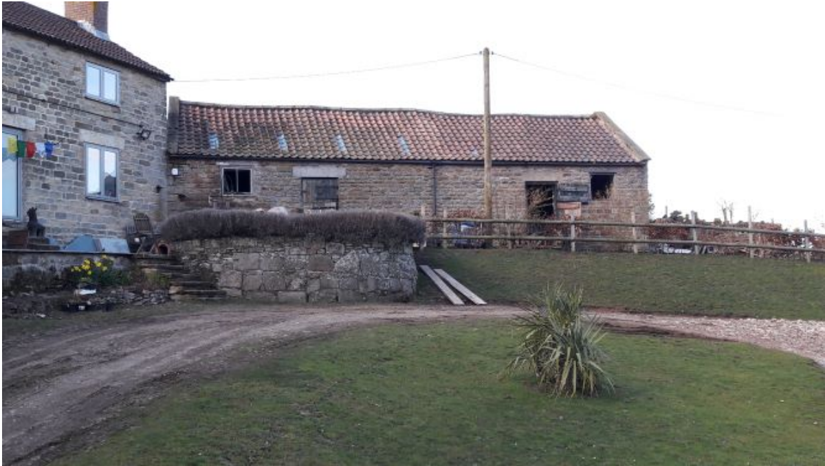
Approach to property showing main house to the left and the stable building to be converted in the centre of the picture. The stable is a single storey stone under pantile building comprising two large stables; each with a stable door and square eaves level window arranged as a mirror image. The site of the proposed greenhouse is to the right of the stable.
