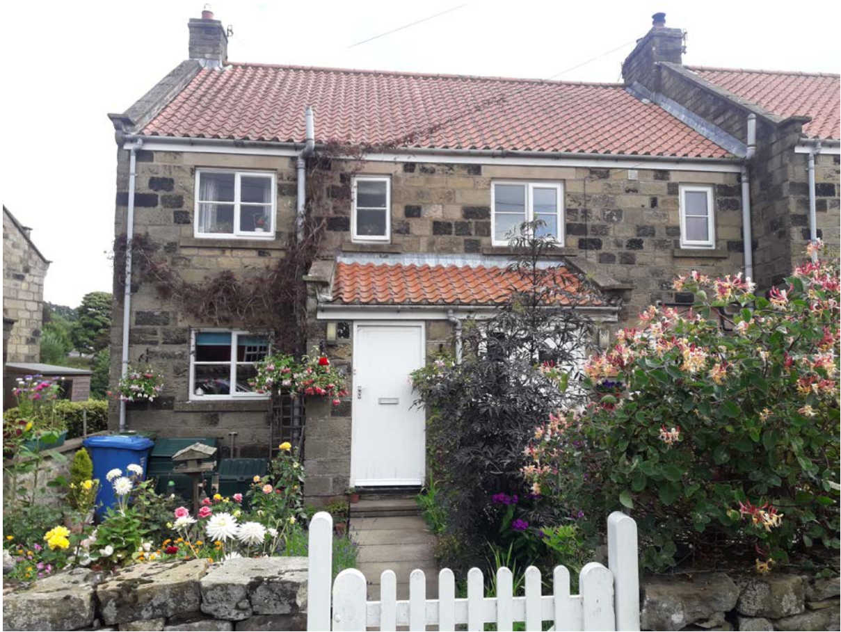
Photo showing front elevation of 6 and 7 Forge Cottages, Lealholm.
