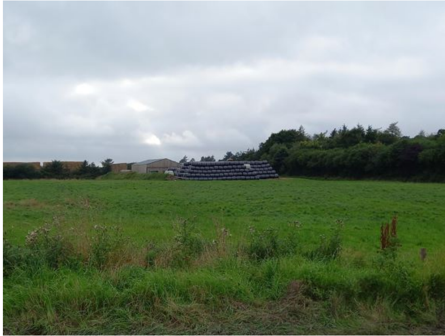
Photograph from site entrance showing modern Yorkshire board building approved in 2018 to the left with stacked wrapped silage bales in the centre. The proposed building is proposed to the right (north) of the 2018 building immediately adjacent the mature tree belt. From this angle, the site is screened from view by the bales.
