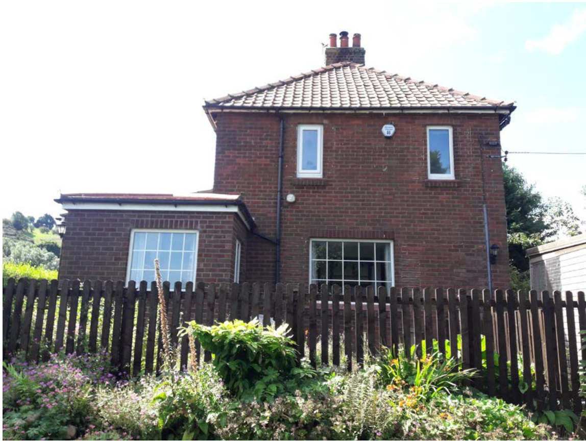
Photo showing side elevation of 161 Coach Road, Sleights.
