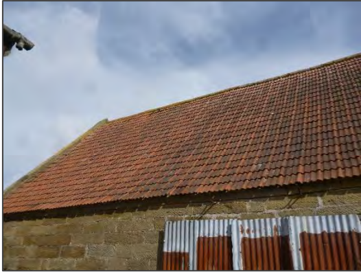
Photo 16: West pitch of roof, 3a.
