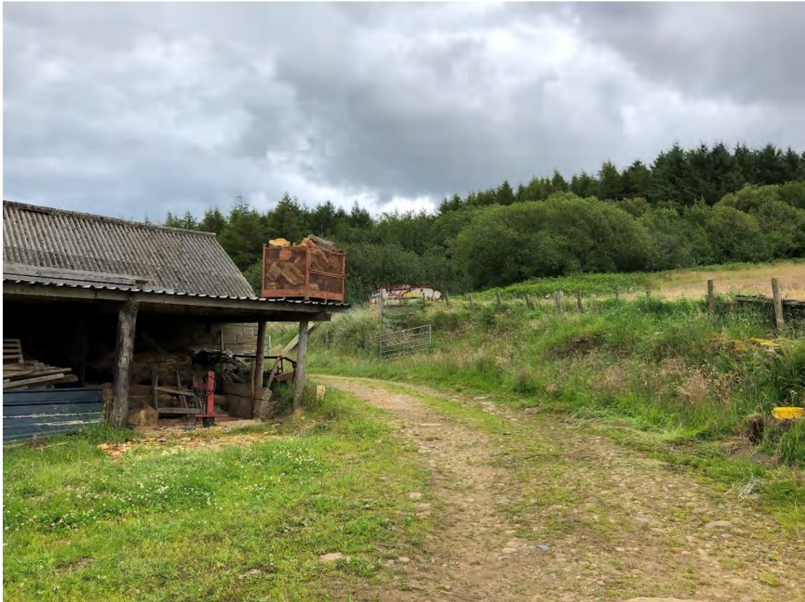
Photograph 3 – West Elevation – South end plus Farm Track
