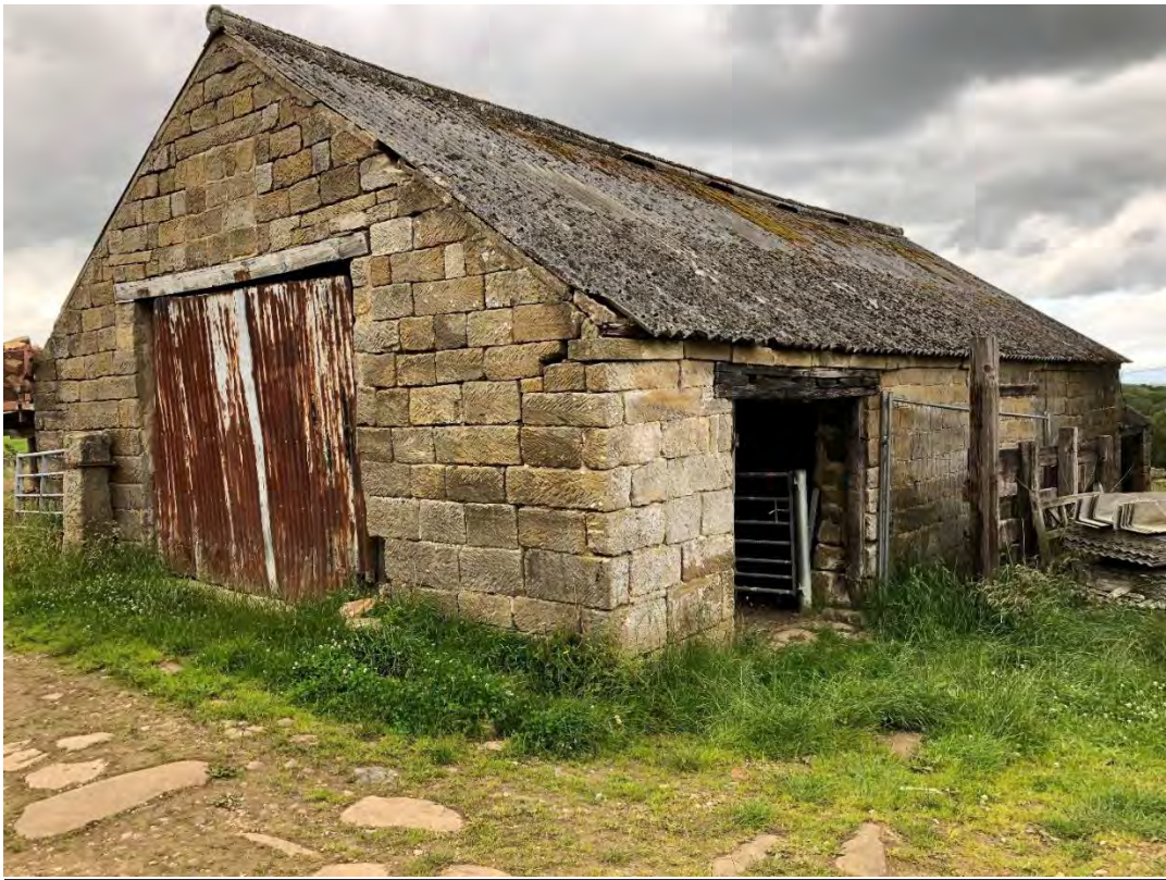
Photograph 1 – Barn B, South Gable and East Side
