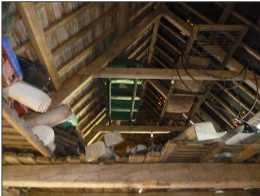
Photo 18: Internal roof 3a.
