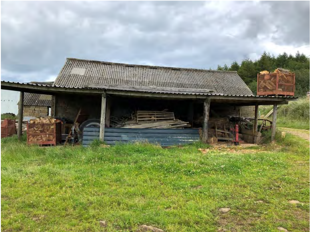
Photograph 2 – West Elevation (Timber Pole Shed)
