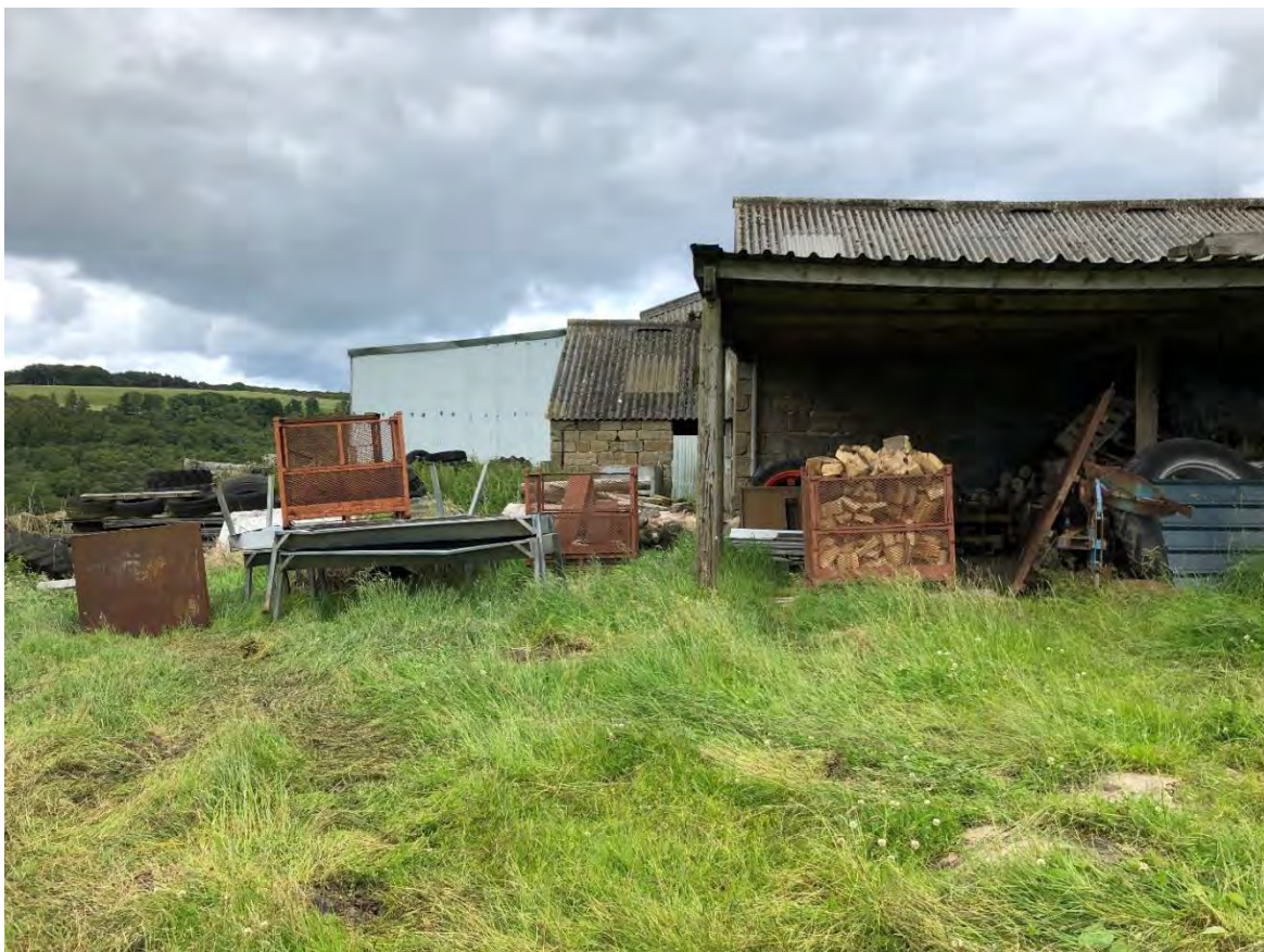
Photograph 4 – West Elevation – North end plus small building
