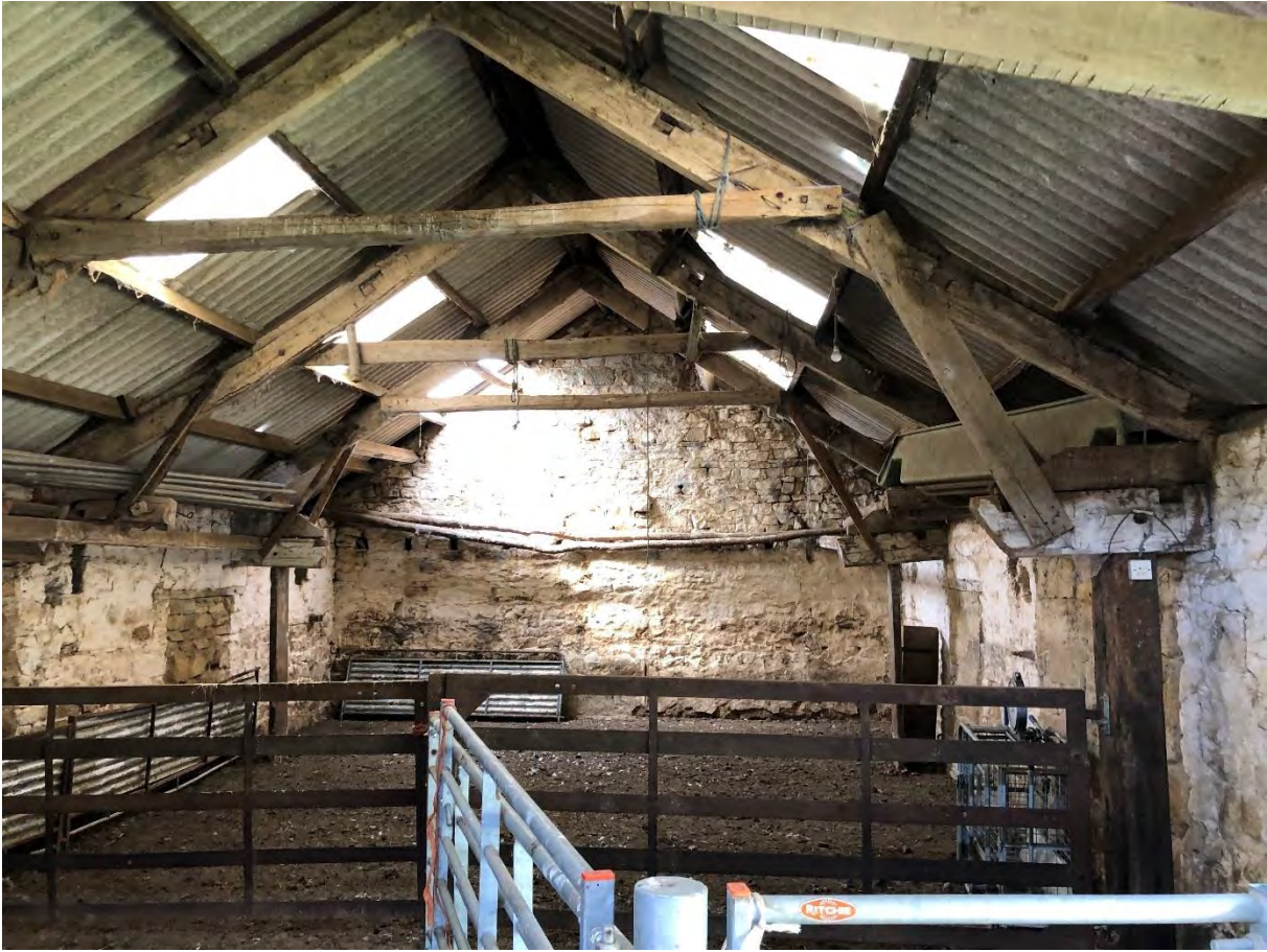
Photograph 11 – Internal looking North
