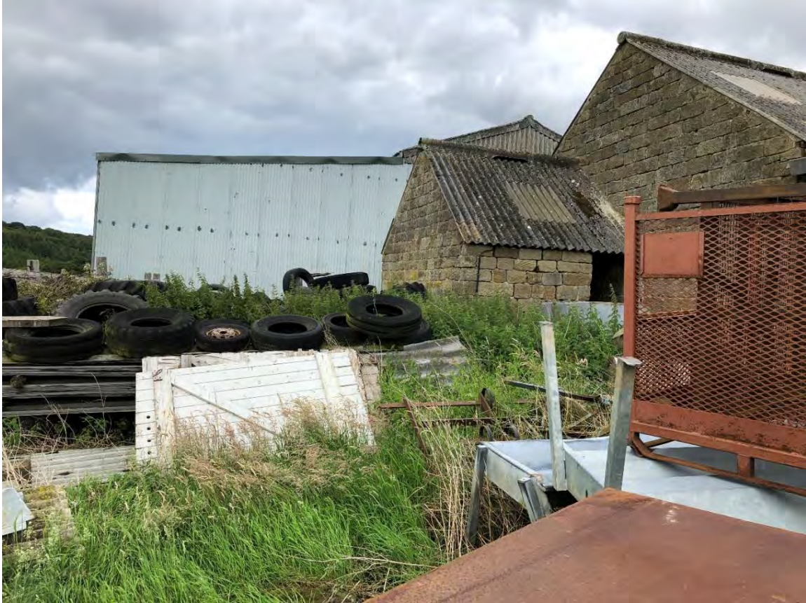
Photograph 5 – North gable and small building
