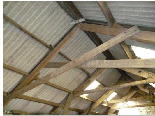
Photo 9: Internal roof, 1a.
