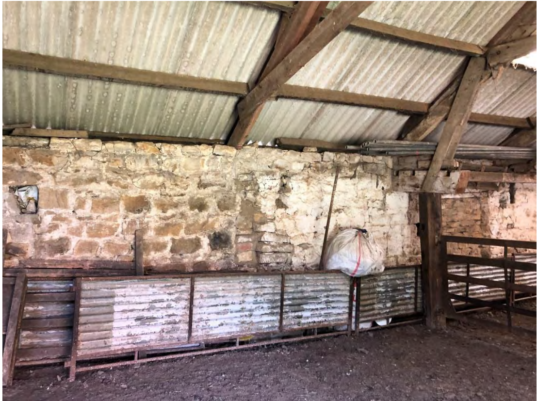
Photograph 10 - Internal looking West
