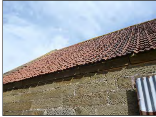
Photo 17: East pitch of roof, 3a.
