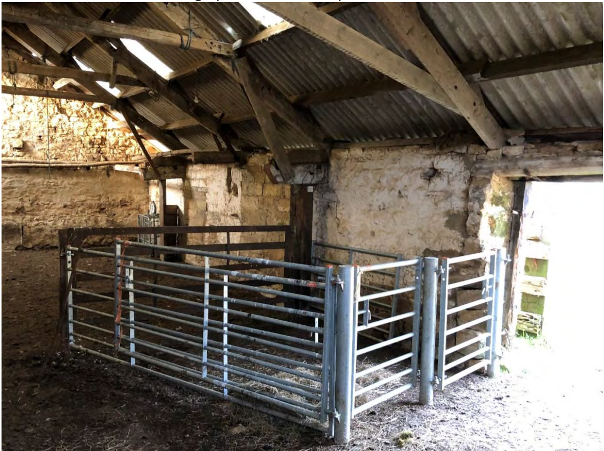
Photograph 14 – East side and part of North Gable
