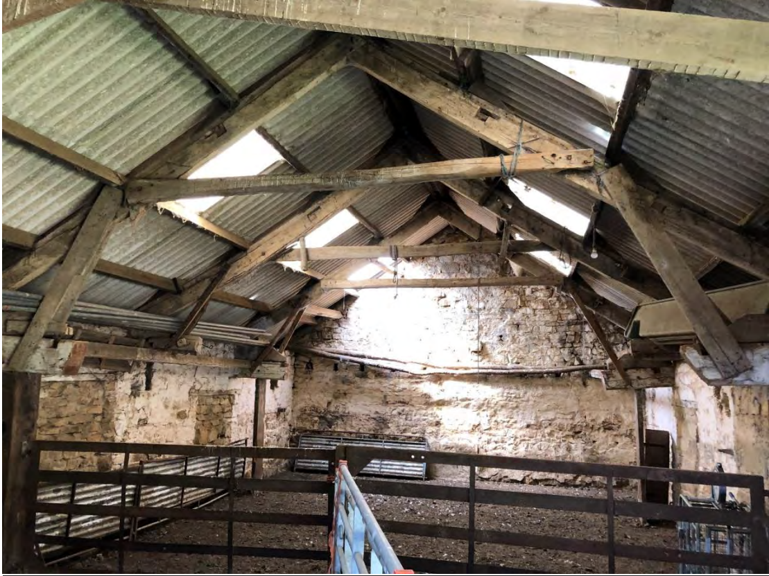
Photograph 9 – Internal looking North
