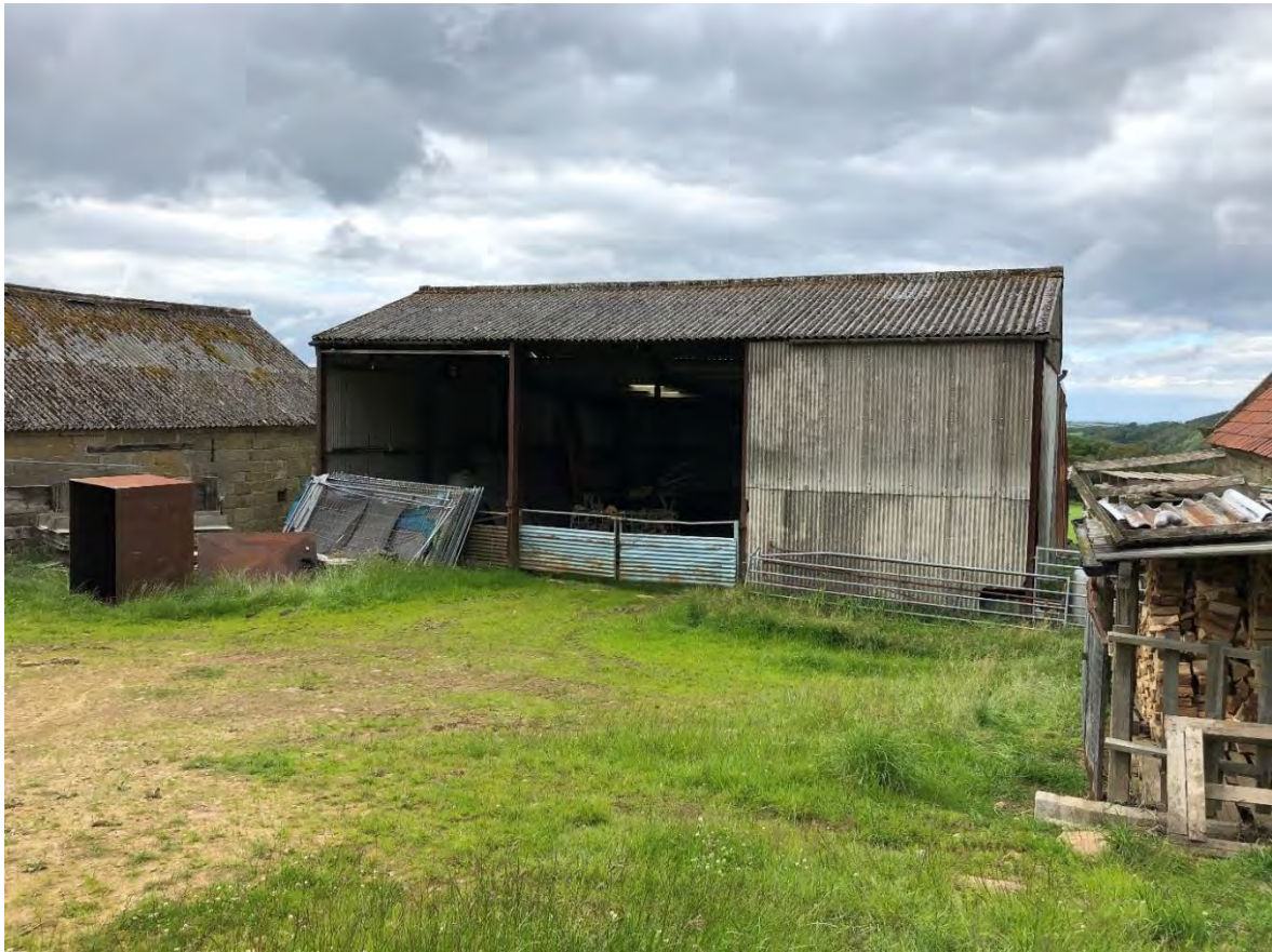
Photograph 8 – Part of East Elevation and Steel Shed
