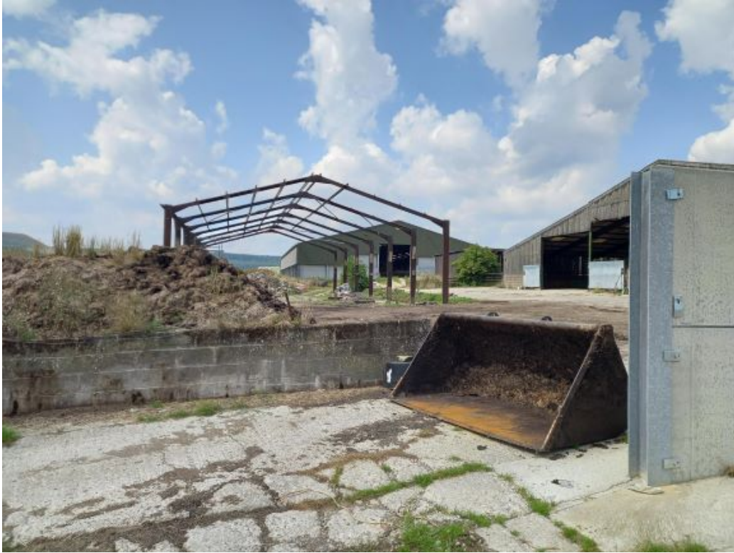
View of development site from within the yard. The steel framework of the former building is seen in the context of the existing large modern sheds.
