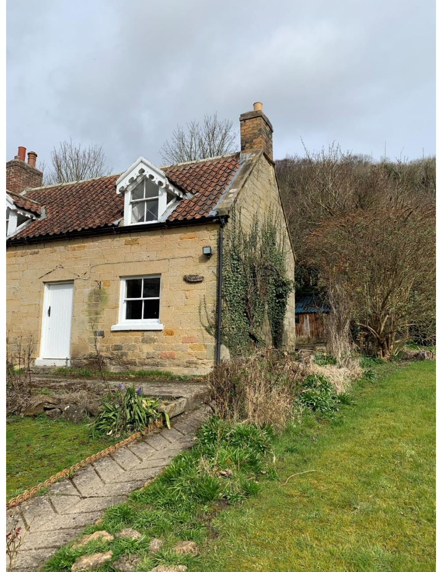
Figure 7 - View towards North of Sunny Crescent
