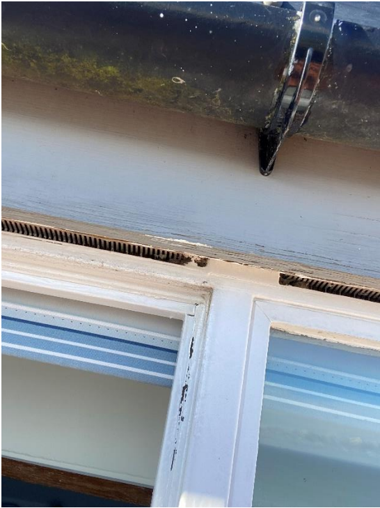
Modern casement window to rear dormer showing sealed glazing to frame
