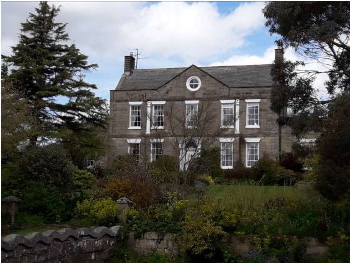
Photo showing front elevation of 34 Main Road, Aislaby.
